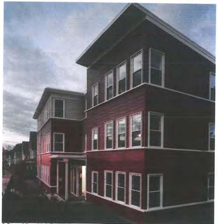
3 Story Nine-Unit Building
