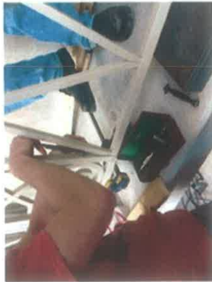
Installing the railing with special tool
