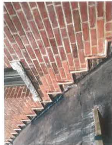
Brick at step flashing
