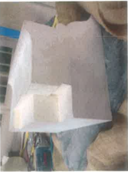
Key way in Dutchman stone to fit down over angle.
