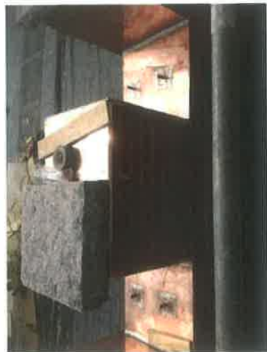
Copper flashing at parapet
