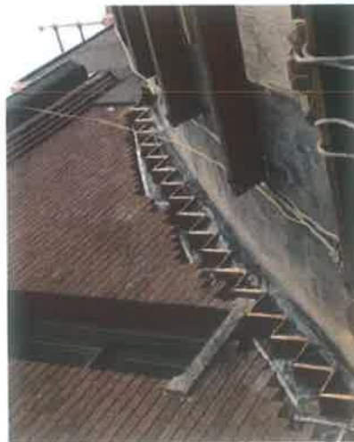
Copper step flashing
