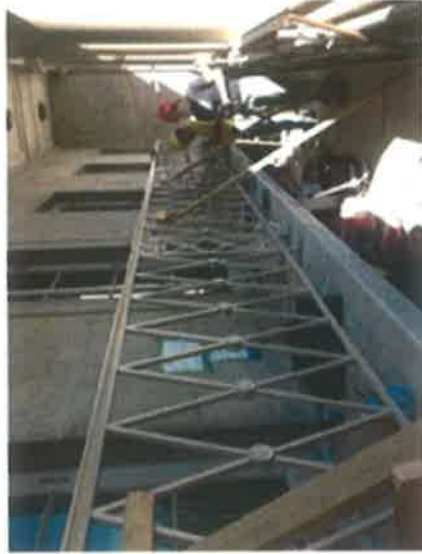
Railing have been plumbed up and braced.
