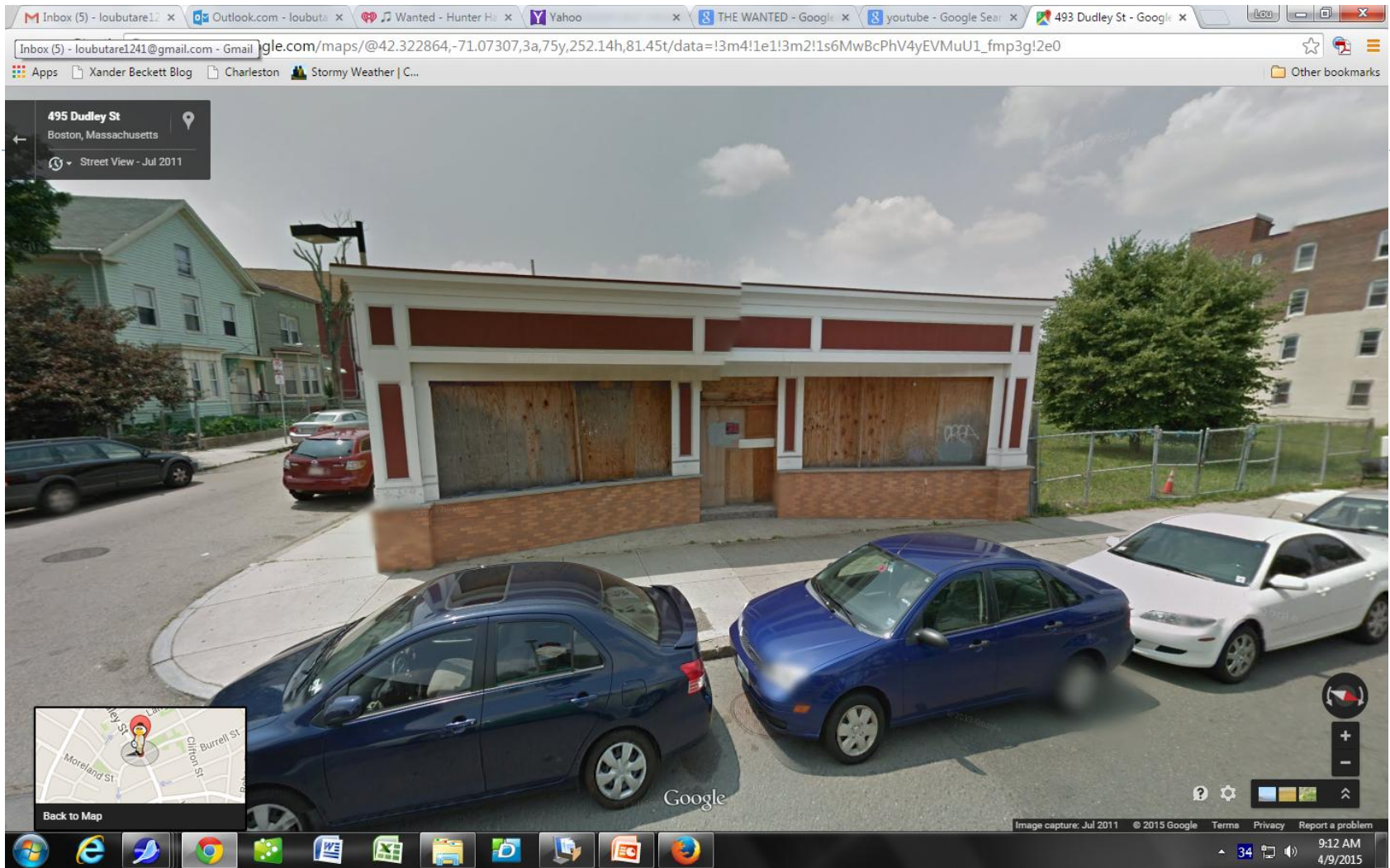
493 DUDLEY STREET – PRIOR TO RENOVATION
