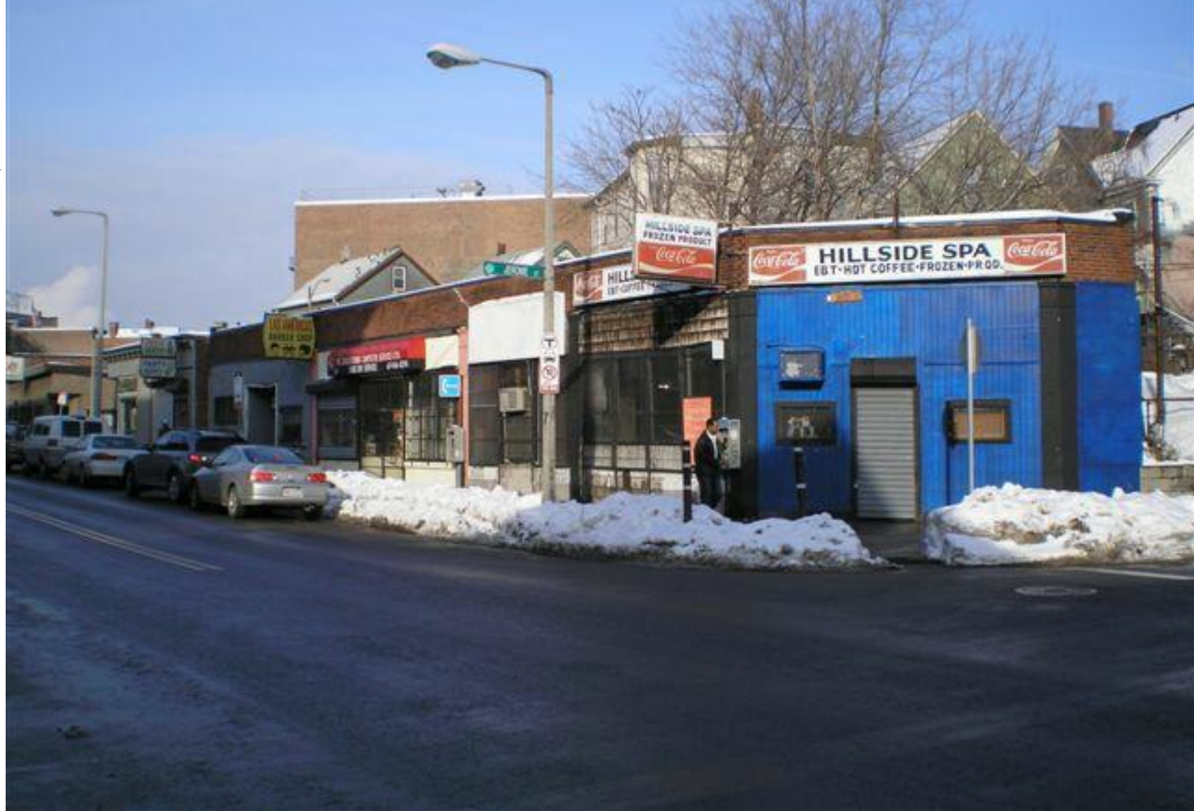
16-24 HANCOCK STREET – PRIOR TO RENOVATION
