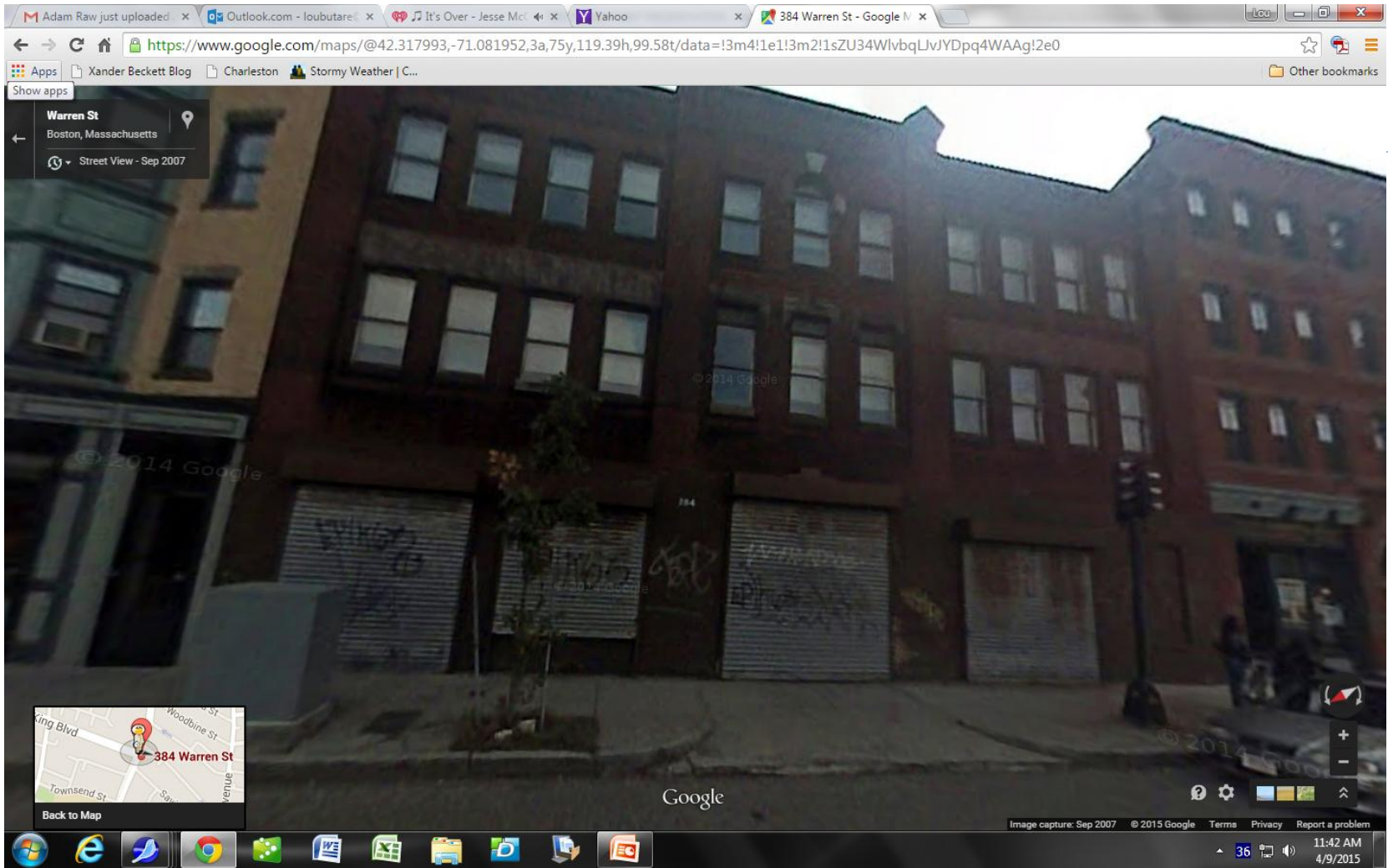
384 WARREN ST. – PRIOR TO RENOVATION
