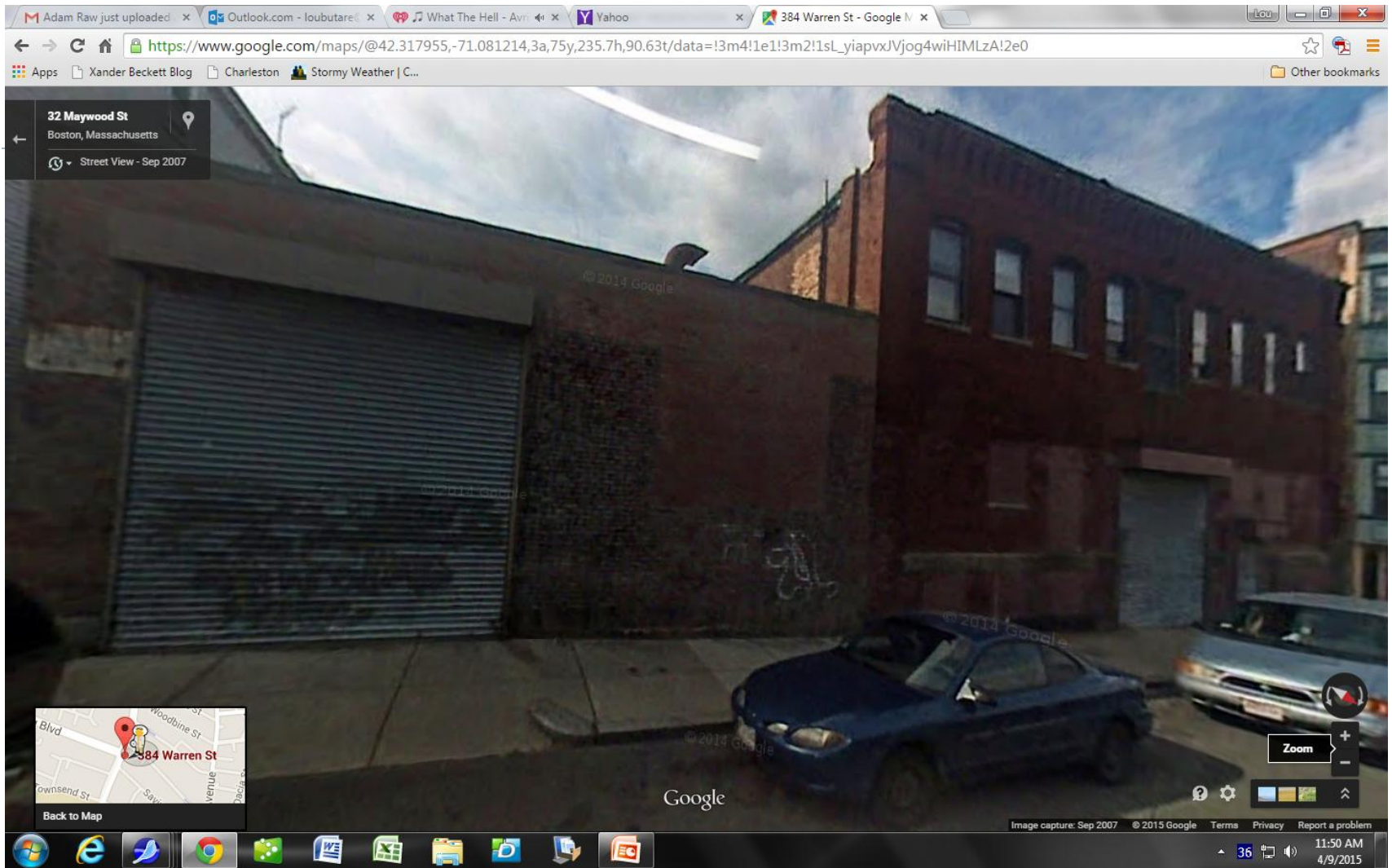
384 WARREN ST. (MAYHEW ST.VIEW) – PRIOR TO RENOVATION
