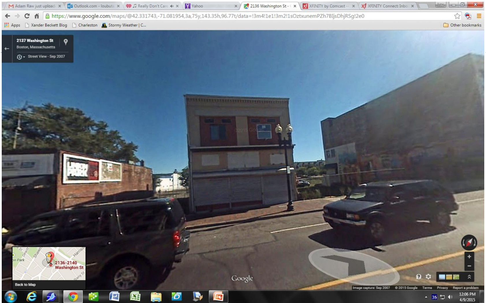
2136 WASHINGTON STREET – PRIOR TO RENOVATION
