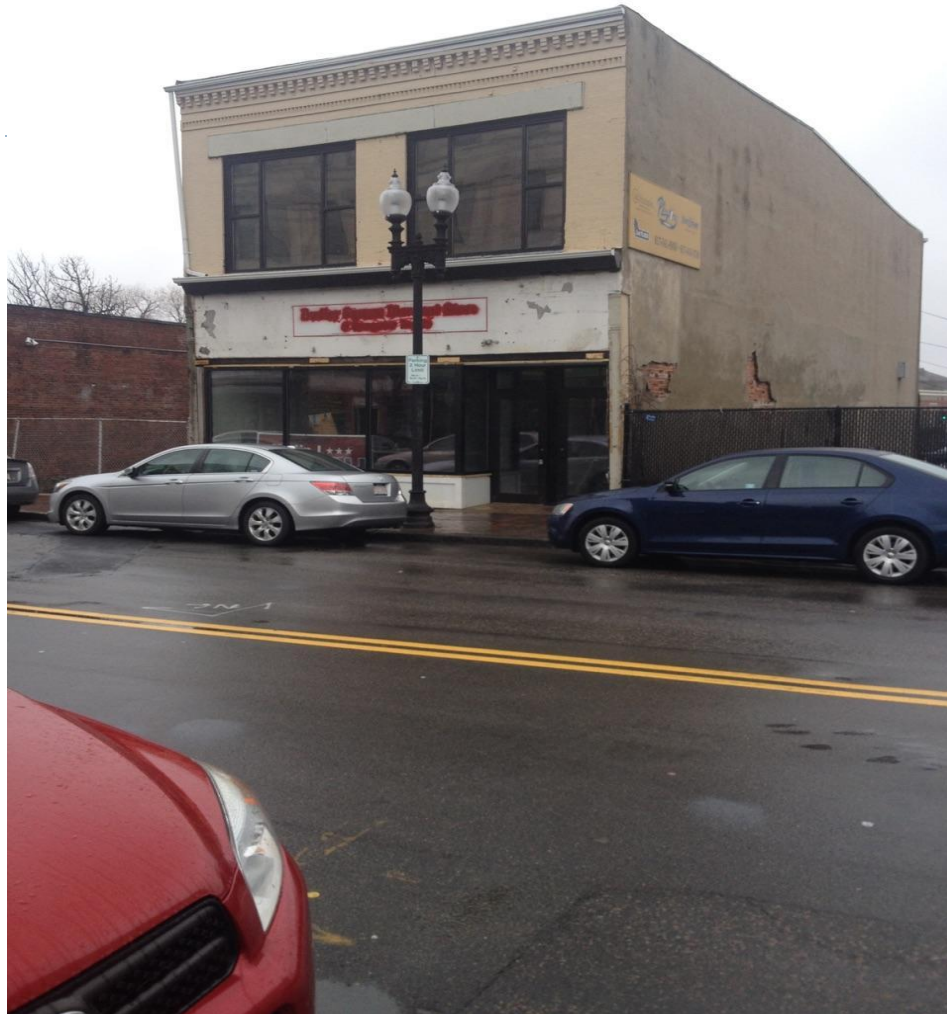
2136 WASHINGTON STREET – TODAY (WORK IN PROGRESS)
