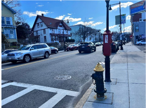
Photo 4: Manholes along Washington Street.
