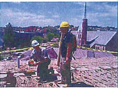
Saint Polycarp Village (Green Roof Installation)
