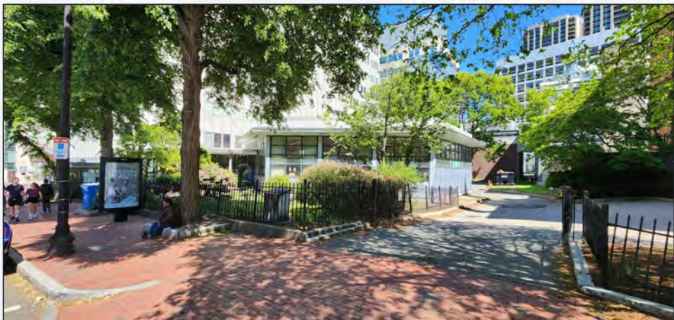
Existing Conditions: West End Library
