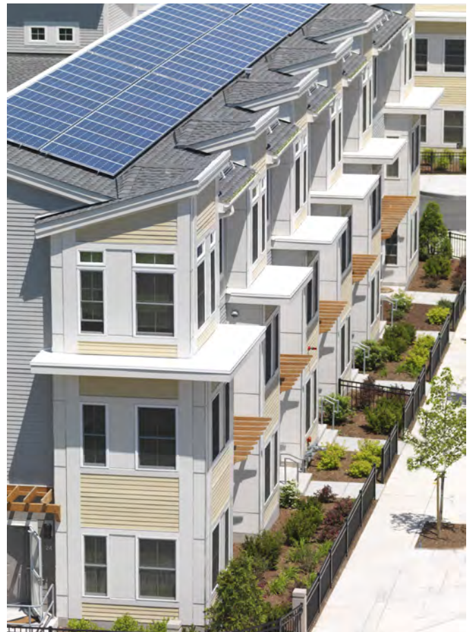
Solar panels on Old Colony BHA housing
