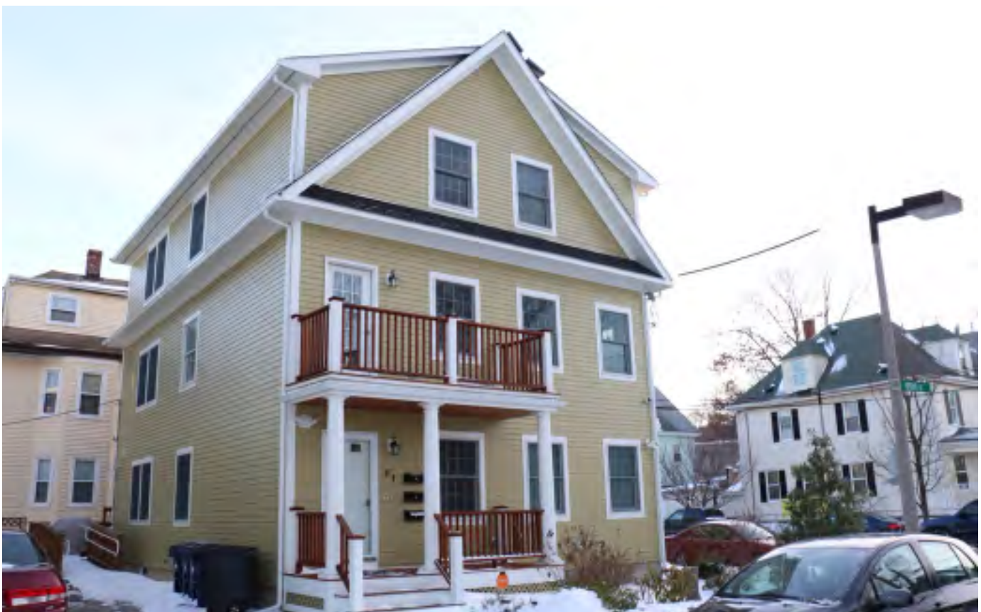
81 Brent St: This LEED Platinum home in Dorchester is 45% more energy efficient than the average home.
