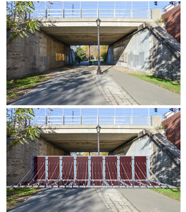
Deployable flood walls, such as the type shown in these renderings of the Greenway under Sumner Street, are installed only when a flood is anticipated. They are otherwise kept in storage.
