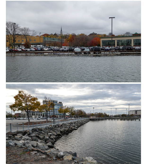
The Schrafft's Center waterfront at 465 Medford Street experienced minor flooding during a King Tide in 2016. With 36 inches of SLR (2070s), these annual high tides will cause extensive flooding.
