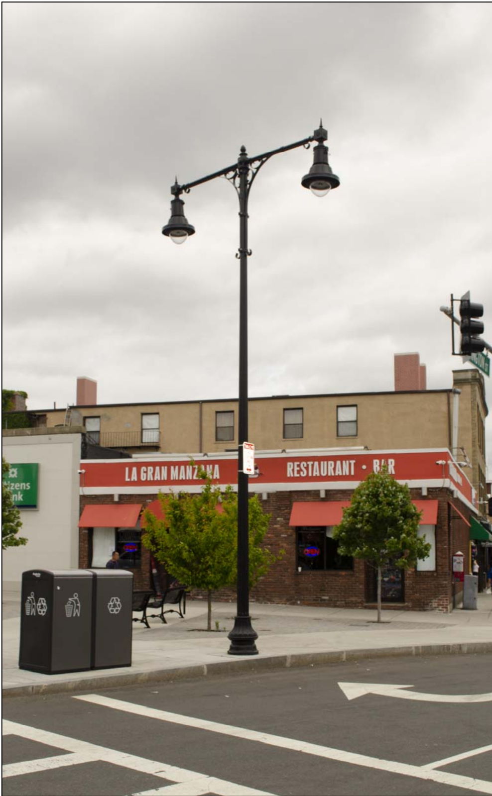
DOUBLE PENDANT LIGHT POLE EXISTING CONDITIONS PHOTOGRAPH - EXHIBIT X-3
