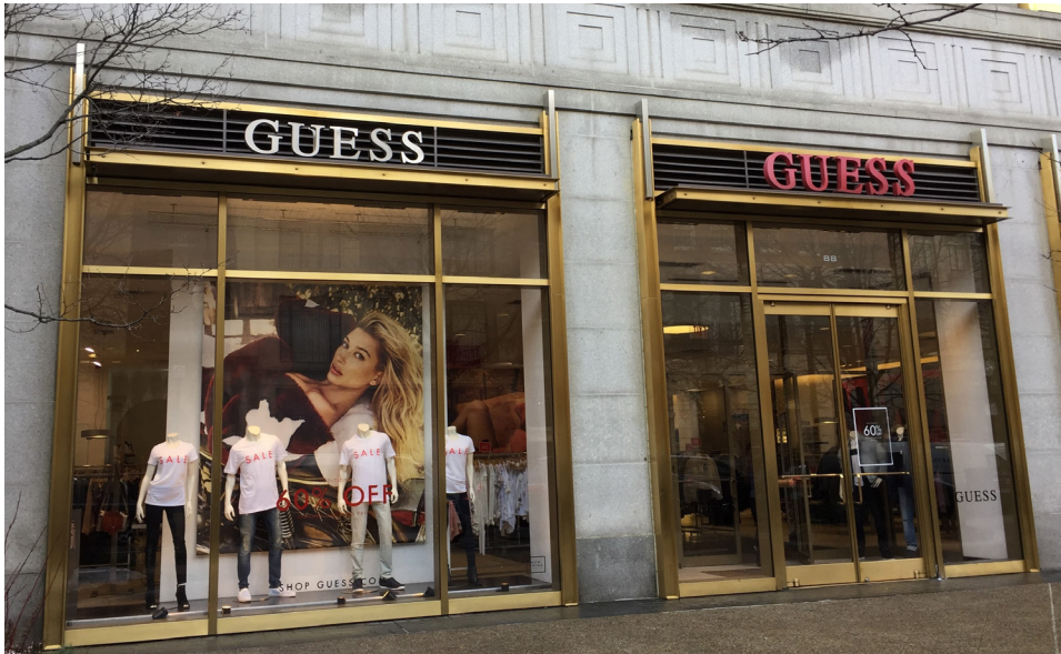
Photo of Existing Condition
