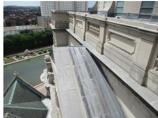
TFCCS – Limestone Coping and Cornices
