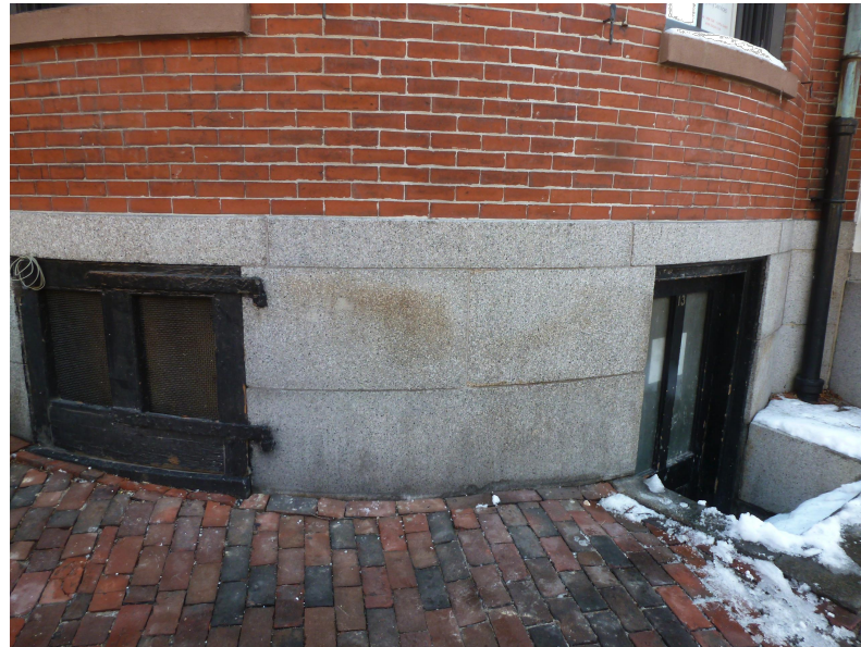
WINDOW & DOOR AT CURVED BAY WEST FACADE
