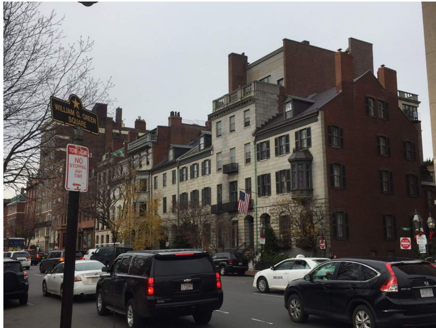
75 Beacon street existing facade
