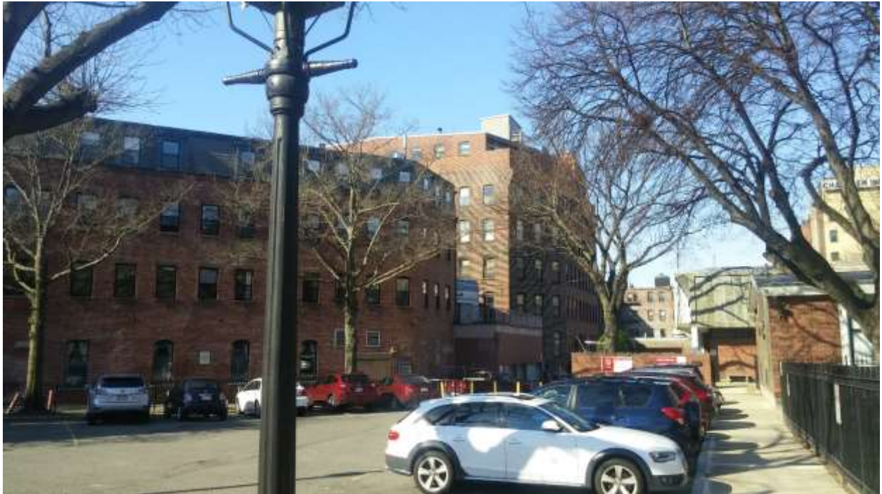
View North West - Rear of Building Parking lot off Tremont Street
