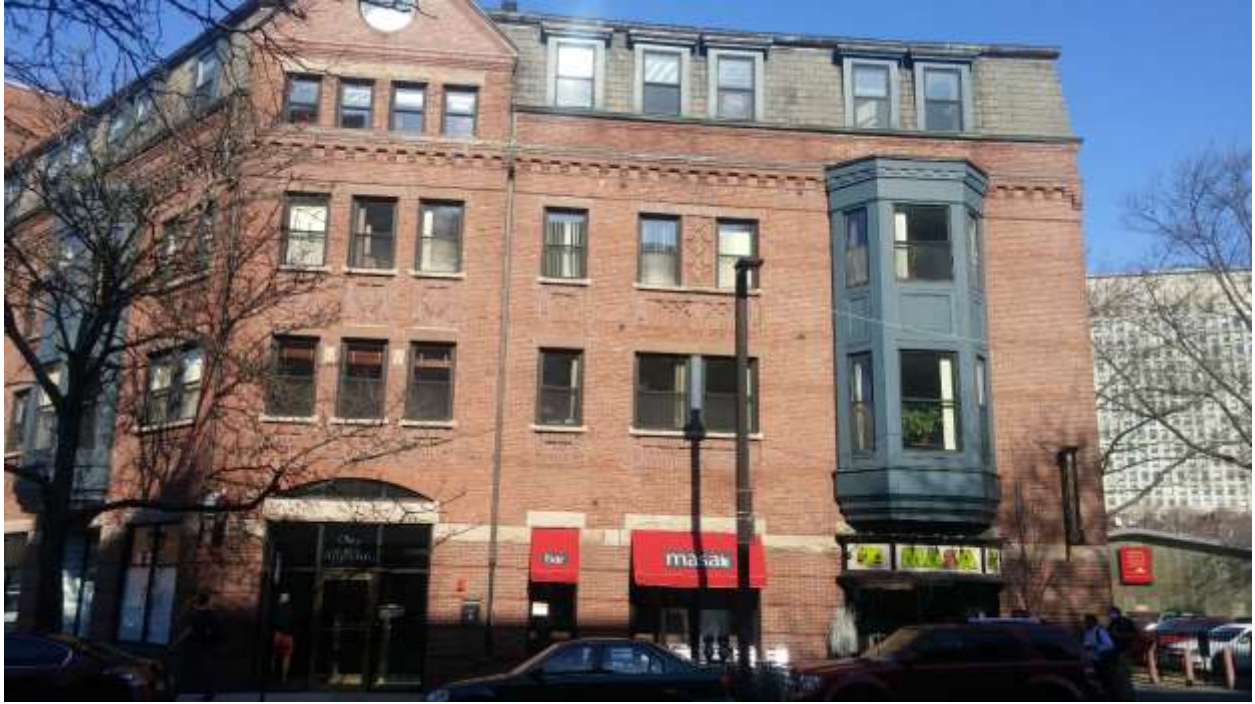
View North Across Tremont Street
