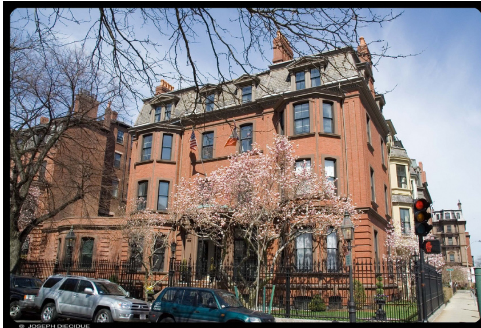
FRENCH CULTURAL CENTER 53 MARLBOROUGH / 300 BERKELEY STREET 6.7.2017
