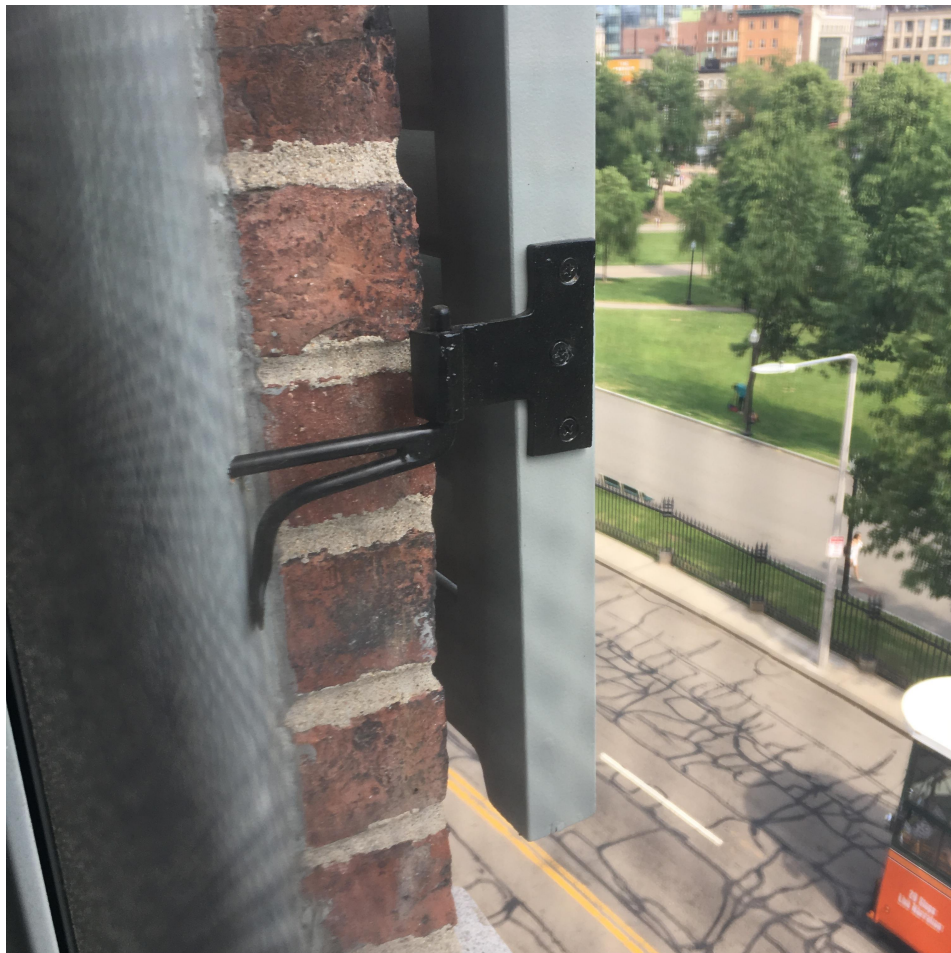
INSTALLED 25 BEACON PINTLE
