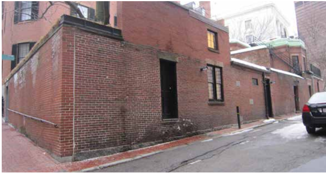
Overall View of Joy Place North Side
