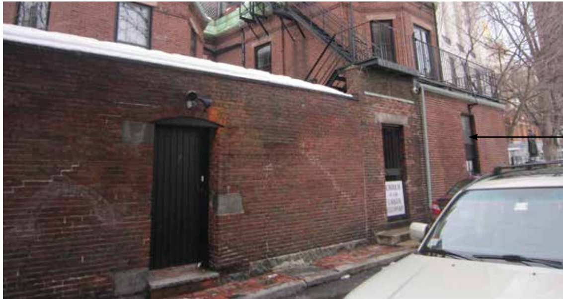
Joy Place North Side - 6 & 7 Mt. Vernon Pl. Prior to Construction
