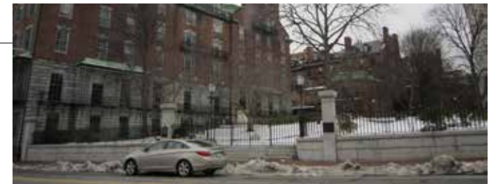
Photo 2A + 2B: View From Beacon Street
