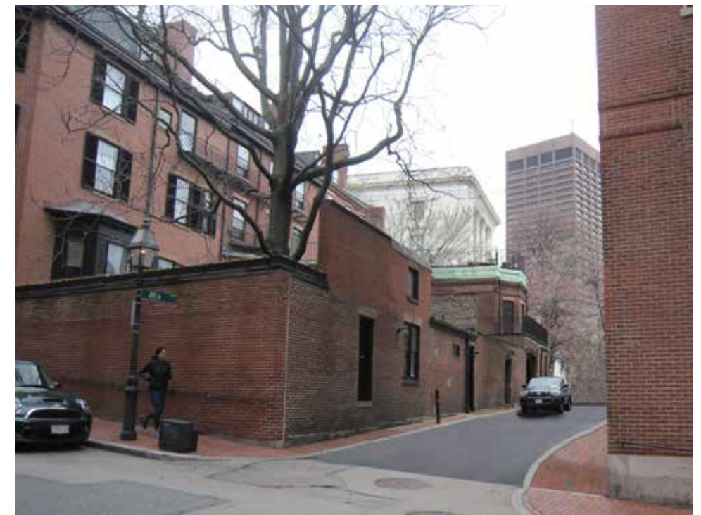
Illustration 8: Proposed View of Joy Place from Joy Street (Fire Escape Removed, Window Added)
