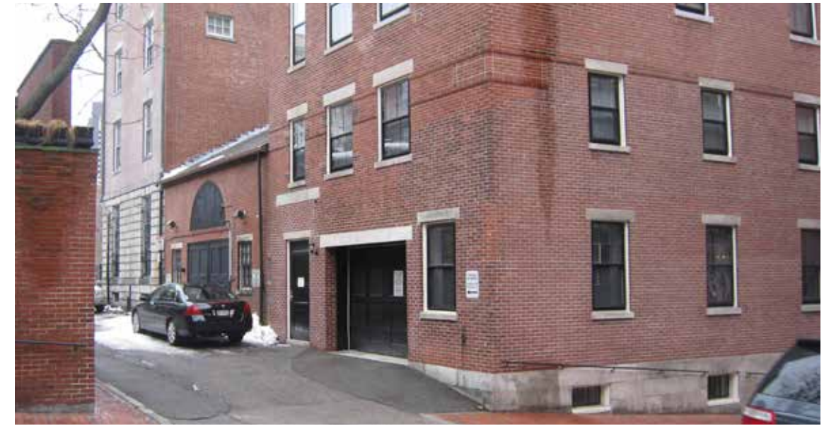
Overall View of Joy Place South Side
