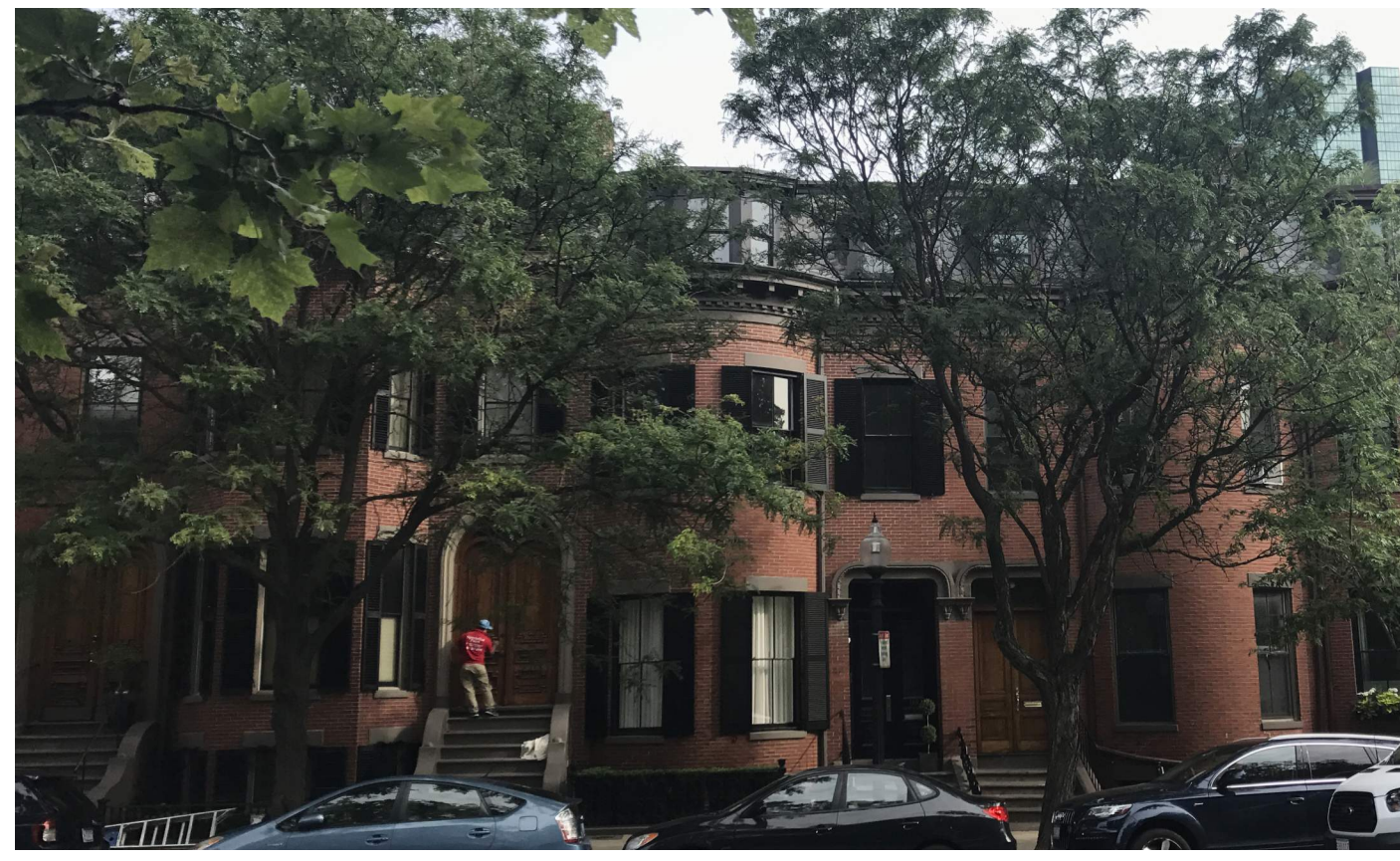
View from across Warren Ave
