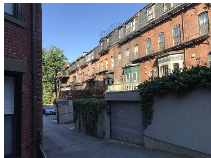
View from rear alley
