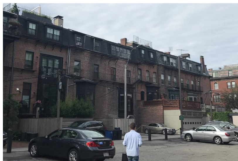
Existing rear facade
