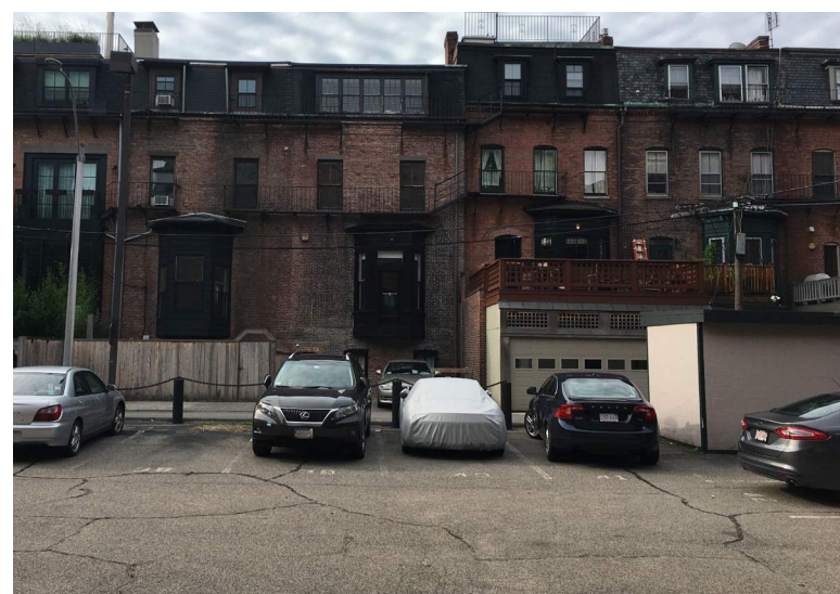
Existing rear facade
