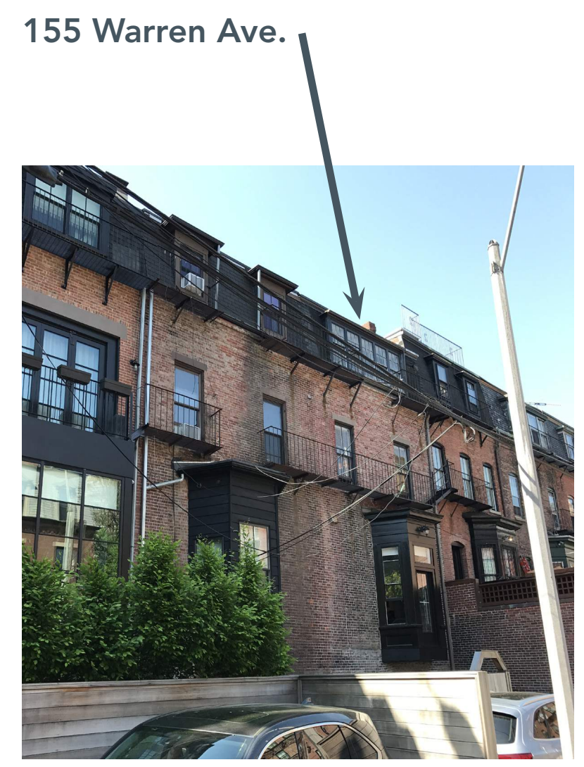
View from rear alley
