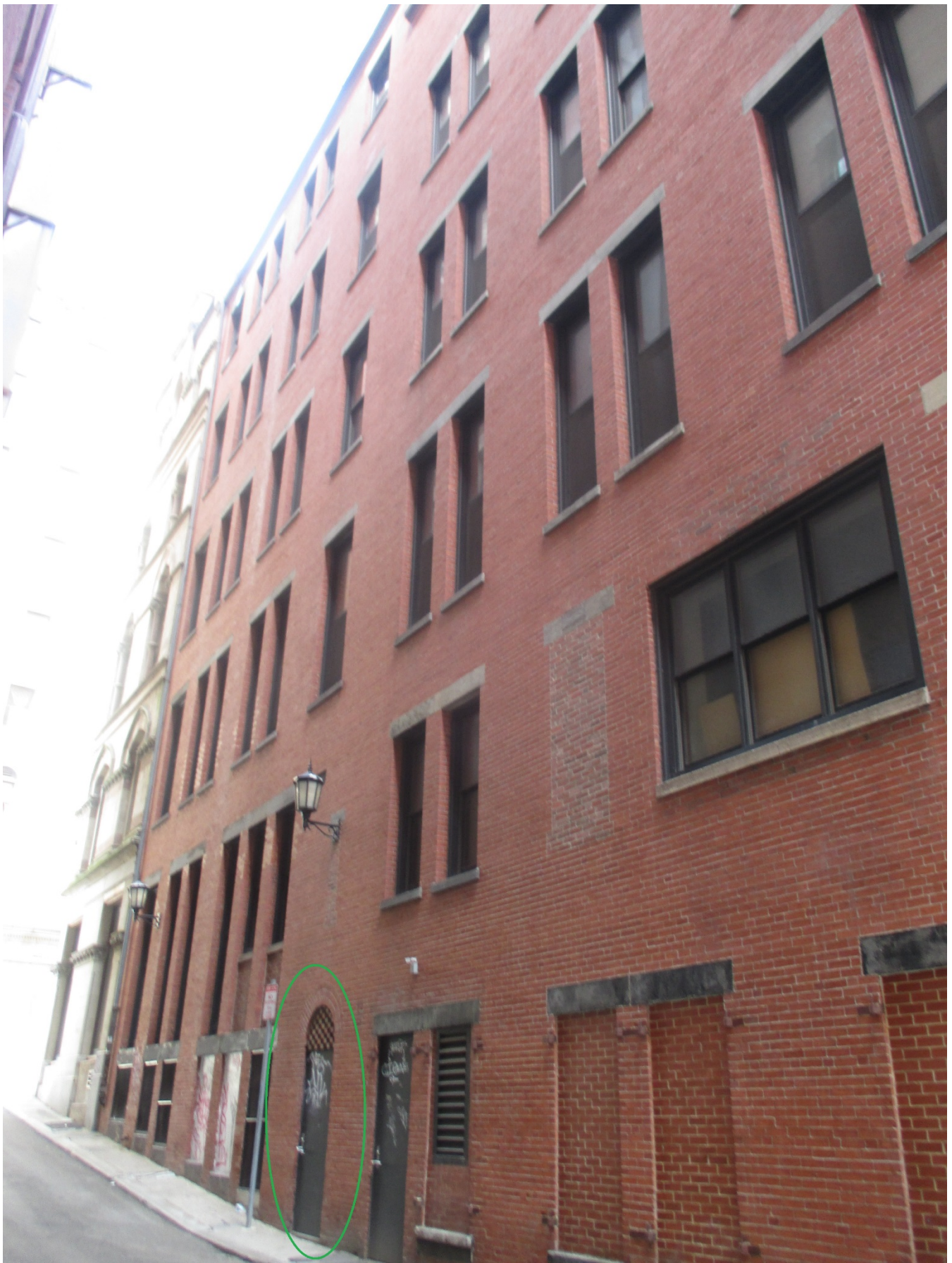
Tamworth Street (west/side) elevation, view northeast
