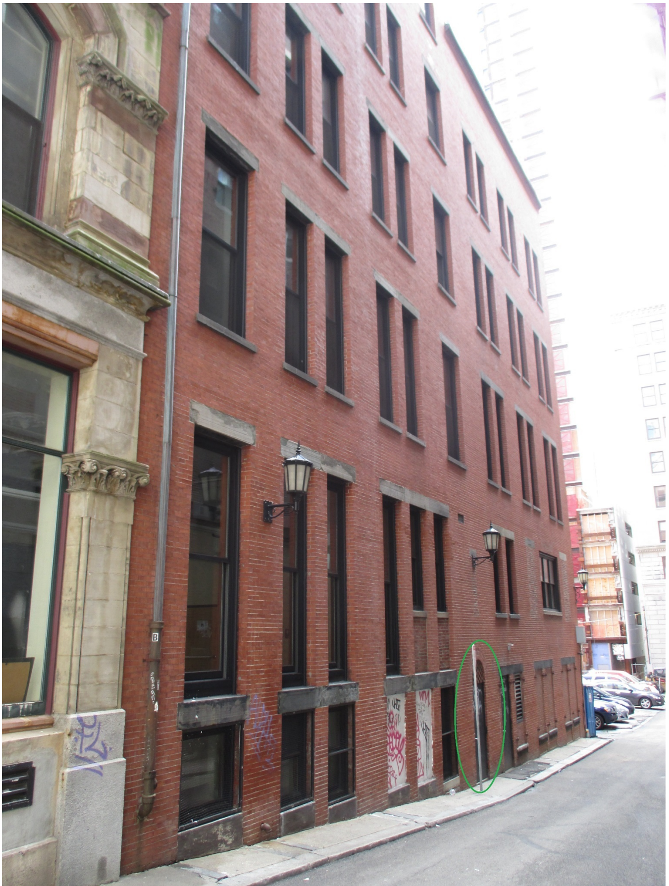
Tamworth Street (west/side) elevation, view southeast
