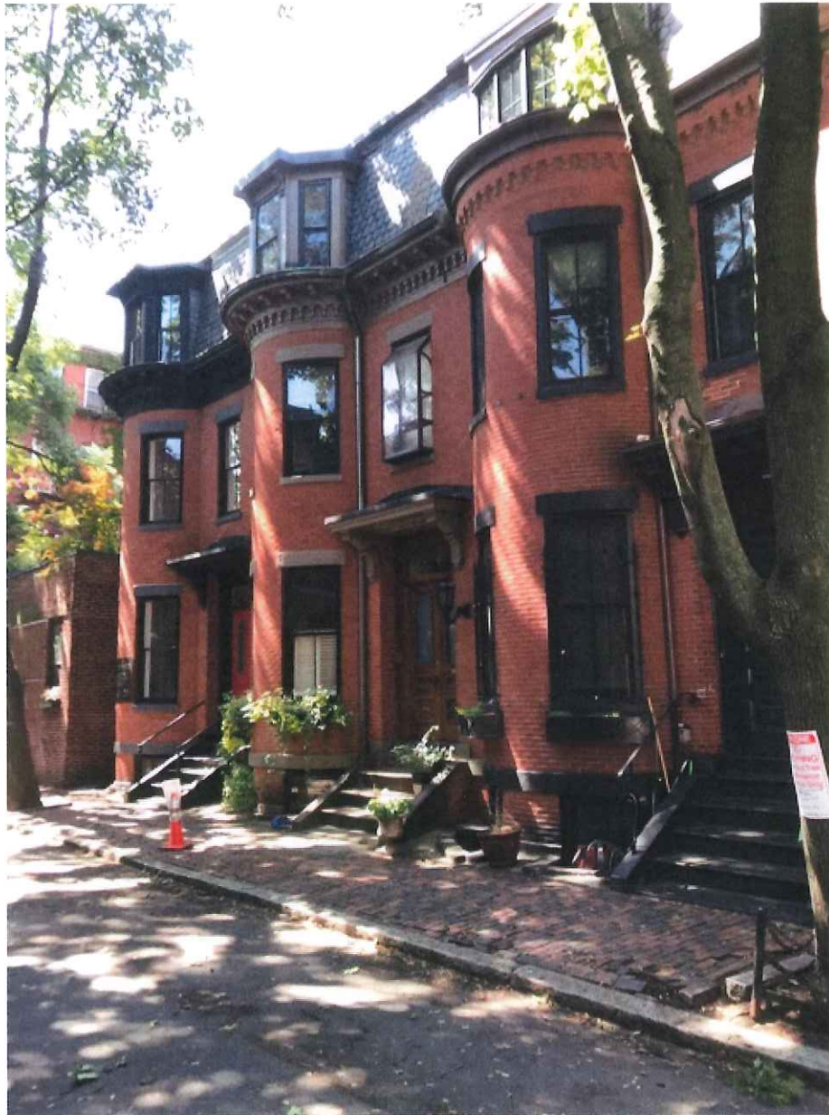
Existing side facade of 2 St. Charles St. looking south towards Chandler St.
