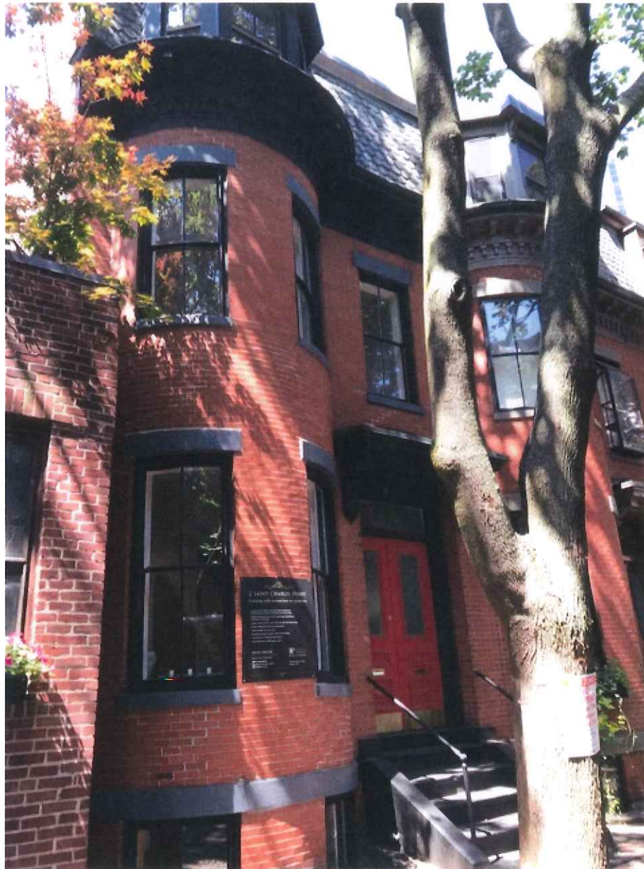
Existing front facade of 2 St. Charles street
