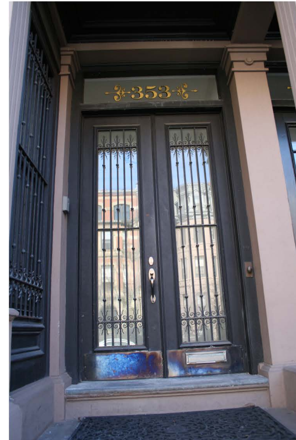
REPLACE EXSITING STAINLESS STEEL HARDWARE (DOOR KNOB AND KICKPLATE) WITH BALDWIN BRASS FIXTURES TO MATCH.
