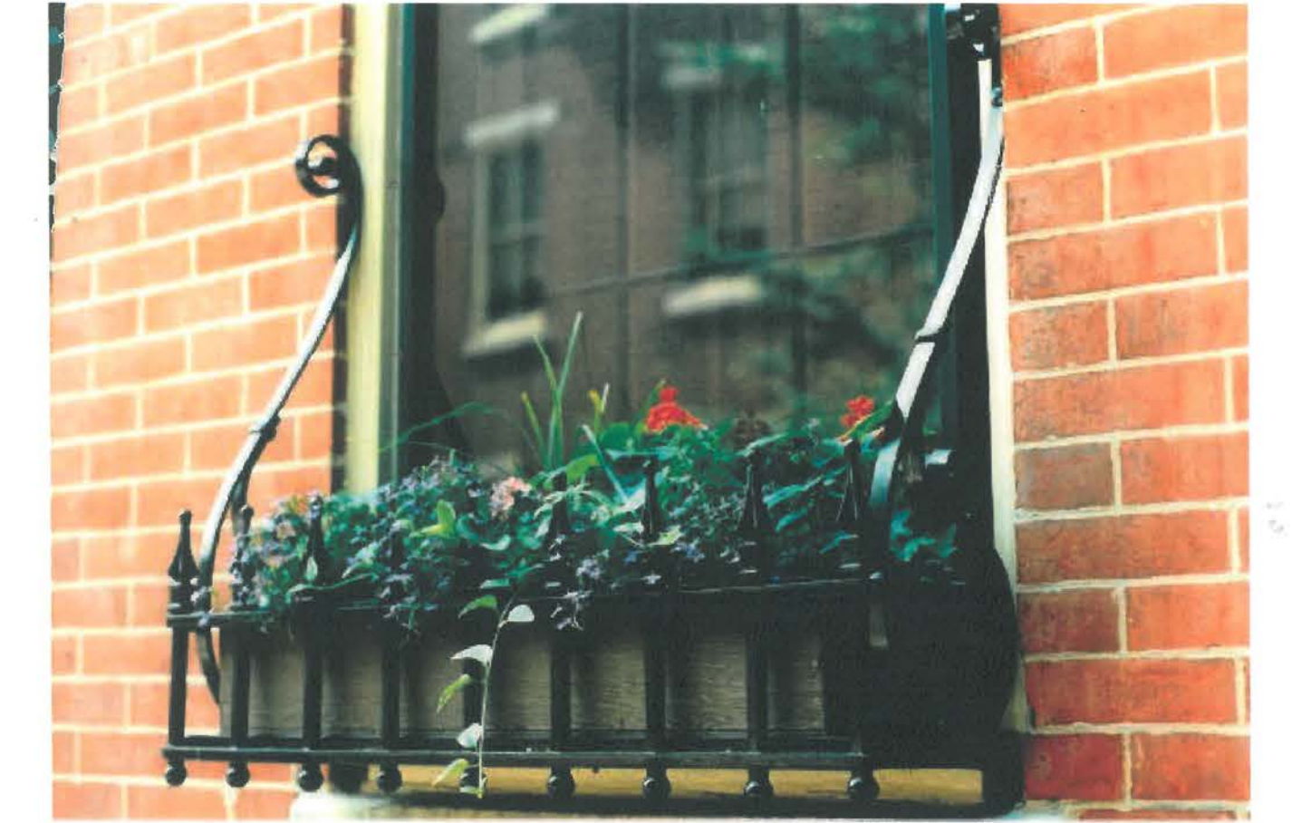
CUSTOM IRON WINDOW BOX HANGER WITH BLACK WINDOW BOX INSERT
