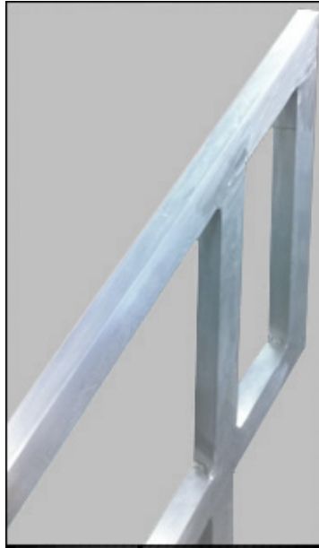
Top of Welded Aluminum Handrail
