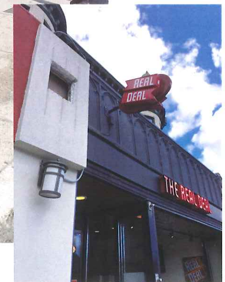
OLD BLADE SIGN LOCATION: 1936 Beacon Street, Boston, Ma 02135
