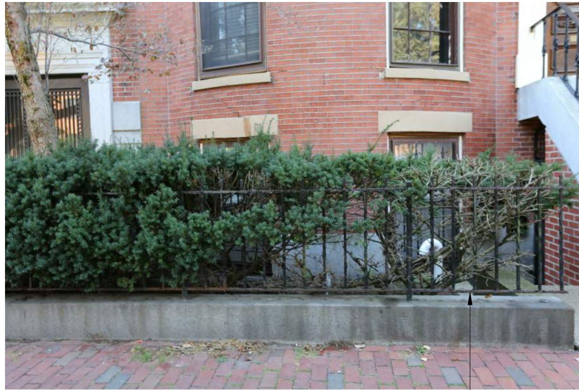
EXISTING RAILING AT PROJECT SITE - 24 UNION PARK
