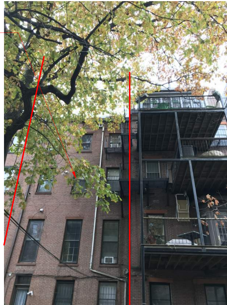
REAR DORMER AT ABUTTING PROPERTY - 22 UNION PARK
