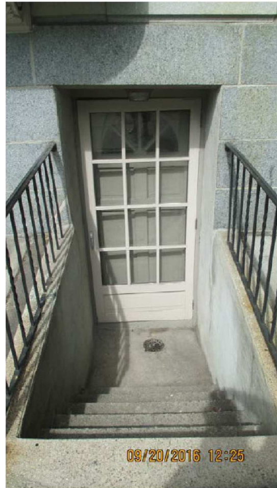
Front basement door, Beacon St.
