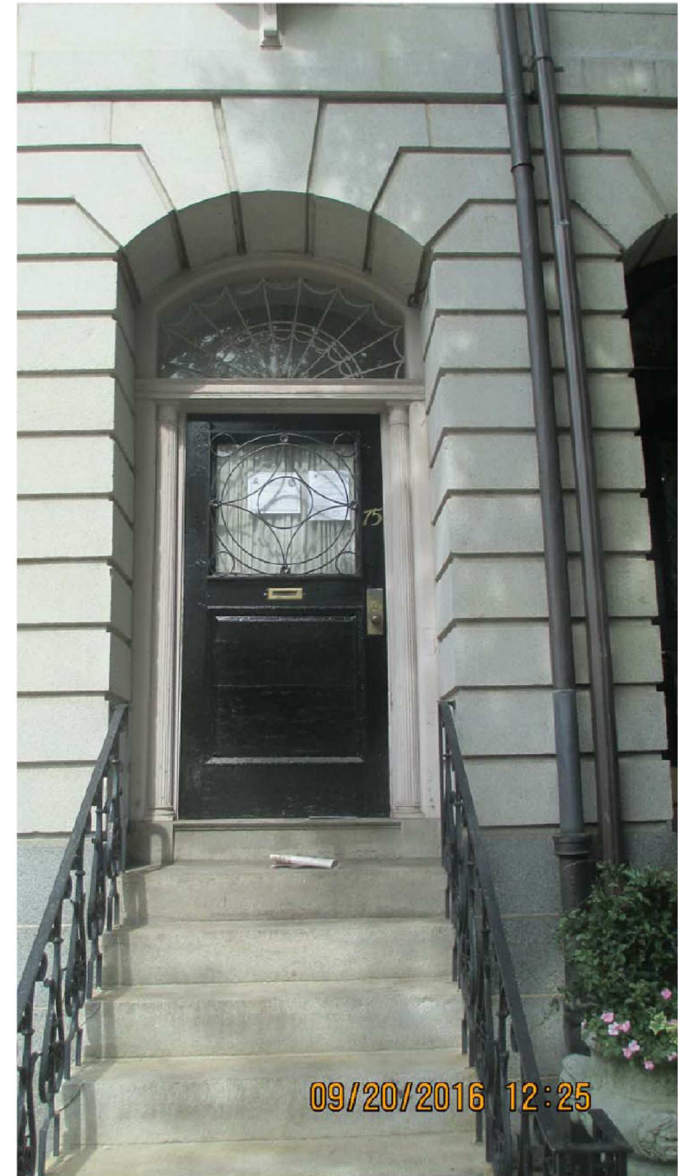
Front door, Beacon St.
