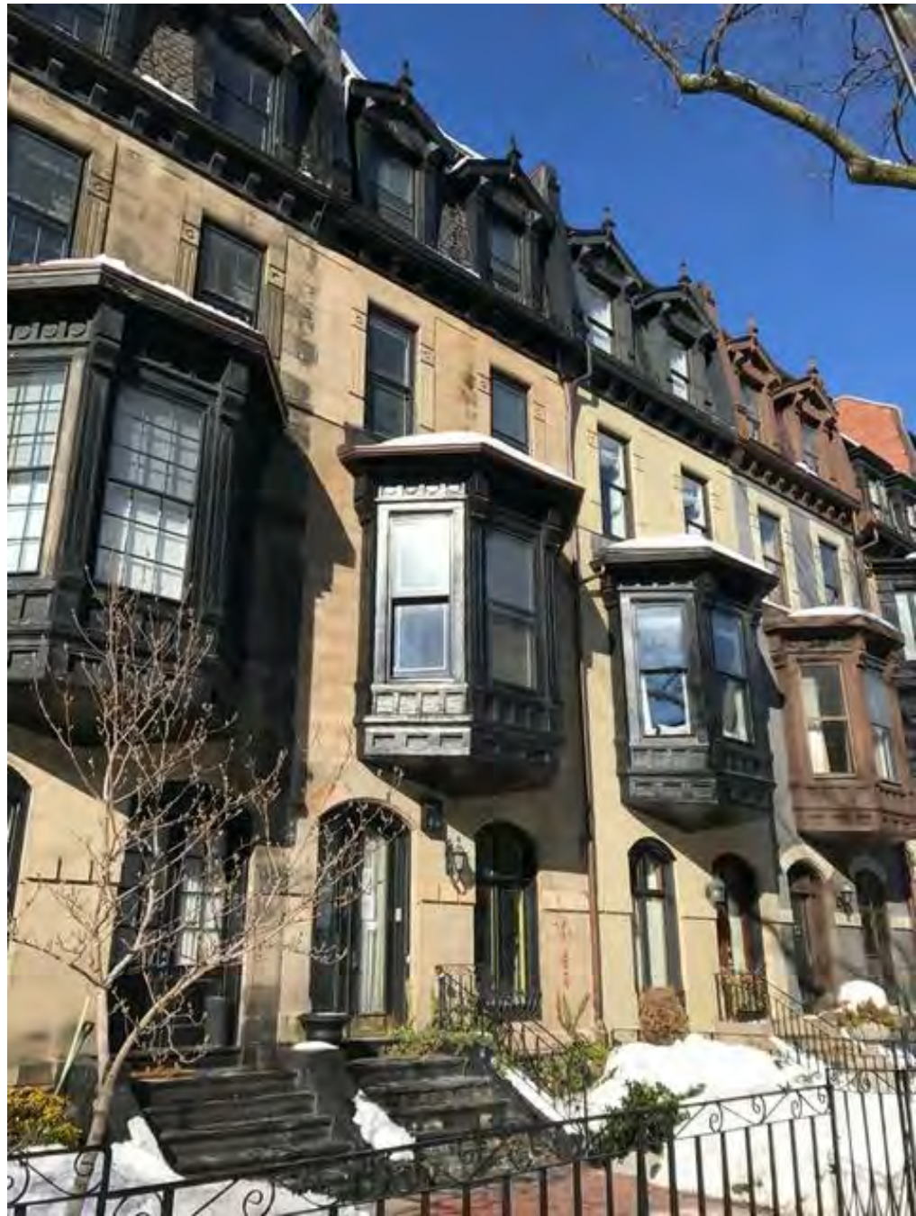
MARLBOROUGH STREET FACADE
