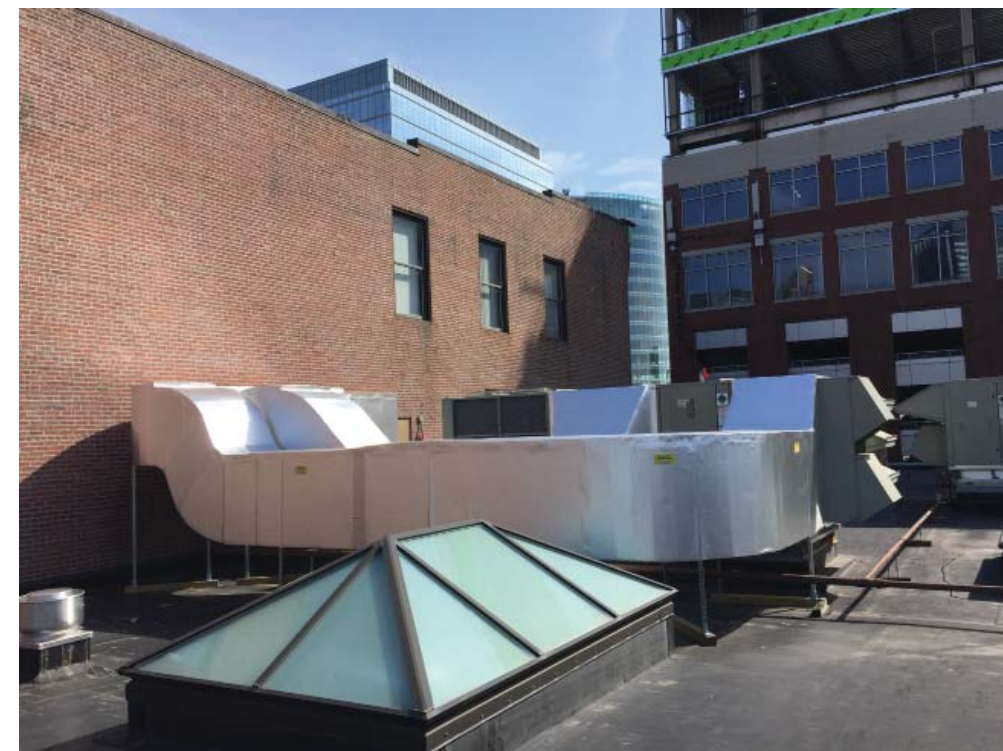
VIEW FROM ROOFTOP- SOUTH
