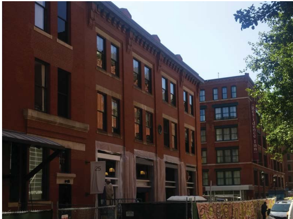
STREET VIEW APPROACHING ON LEFT
