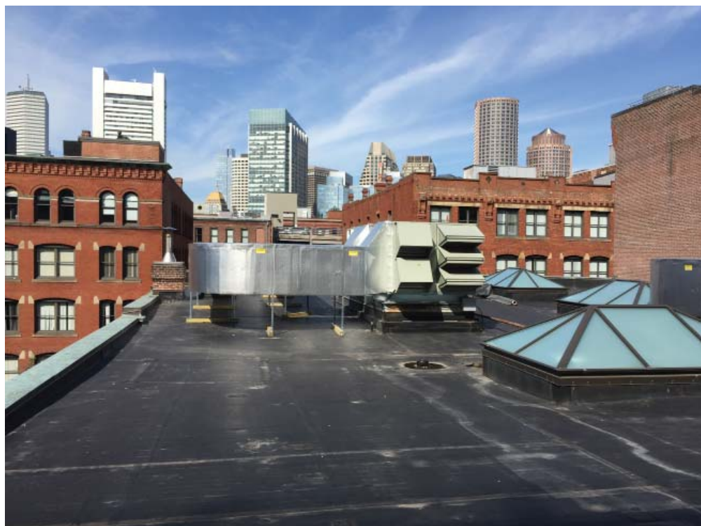
VIEW FROM ROOFTOP- NORTH
