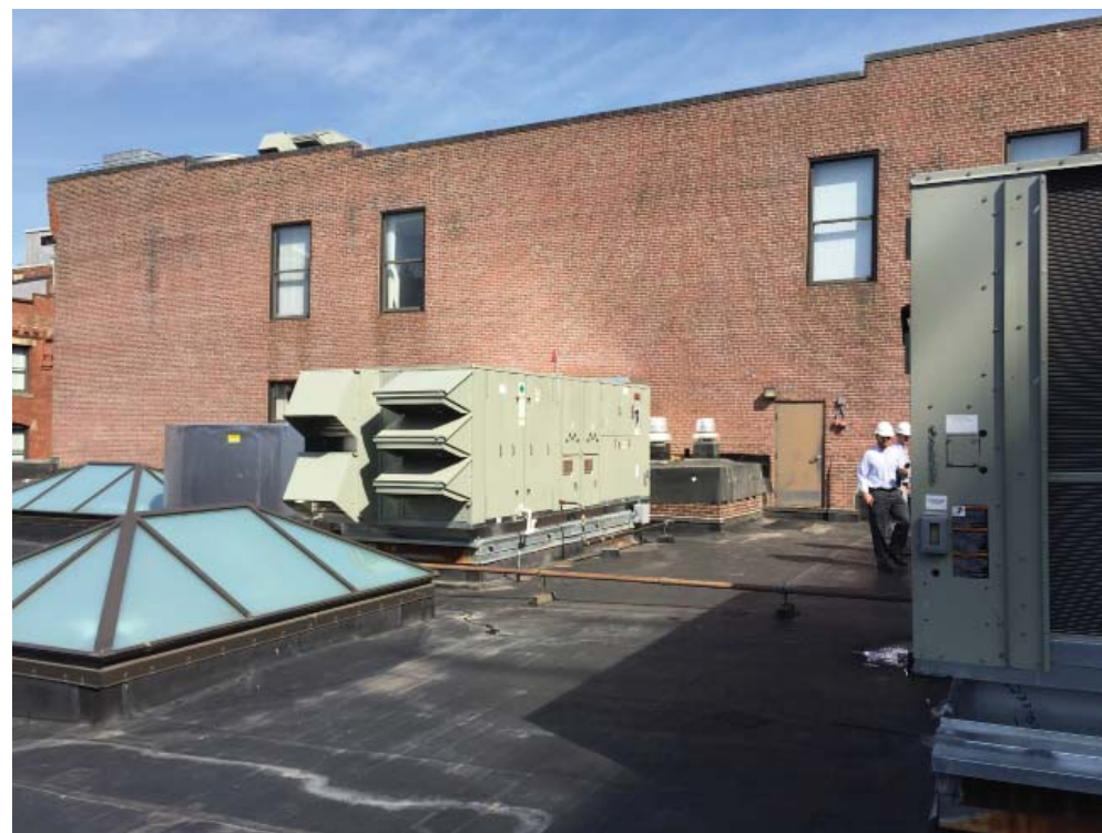
VIEW FROM ROOFTOP- EAST
