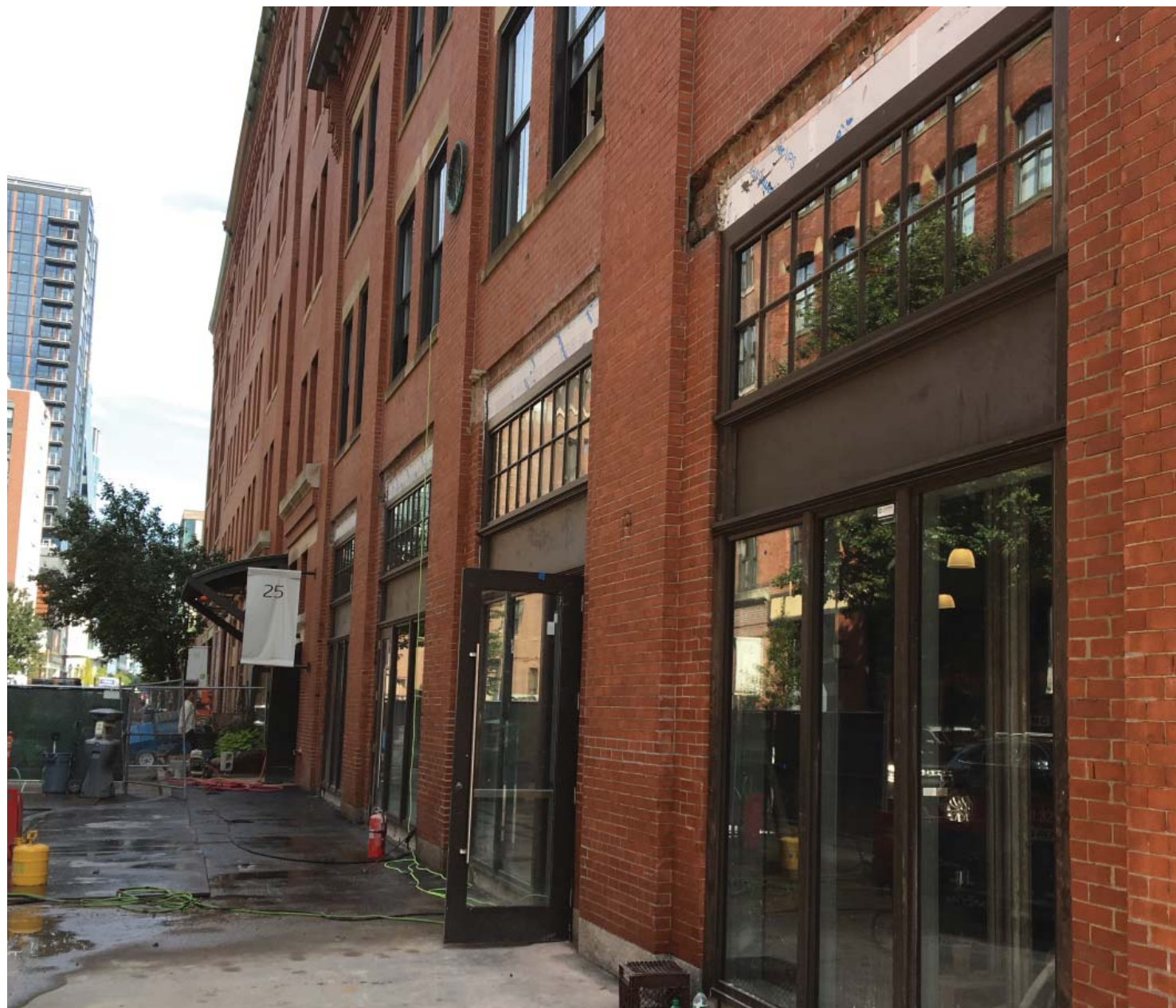
VIEW ALONG THOMSON PLACE
