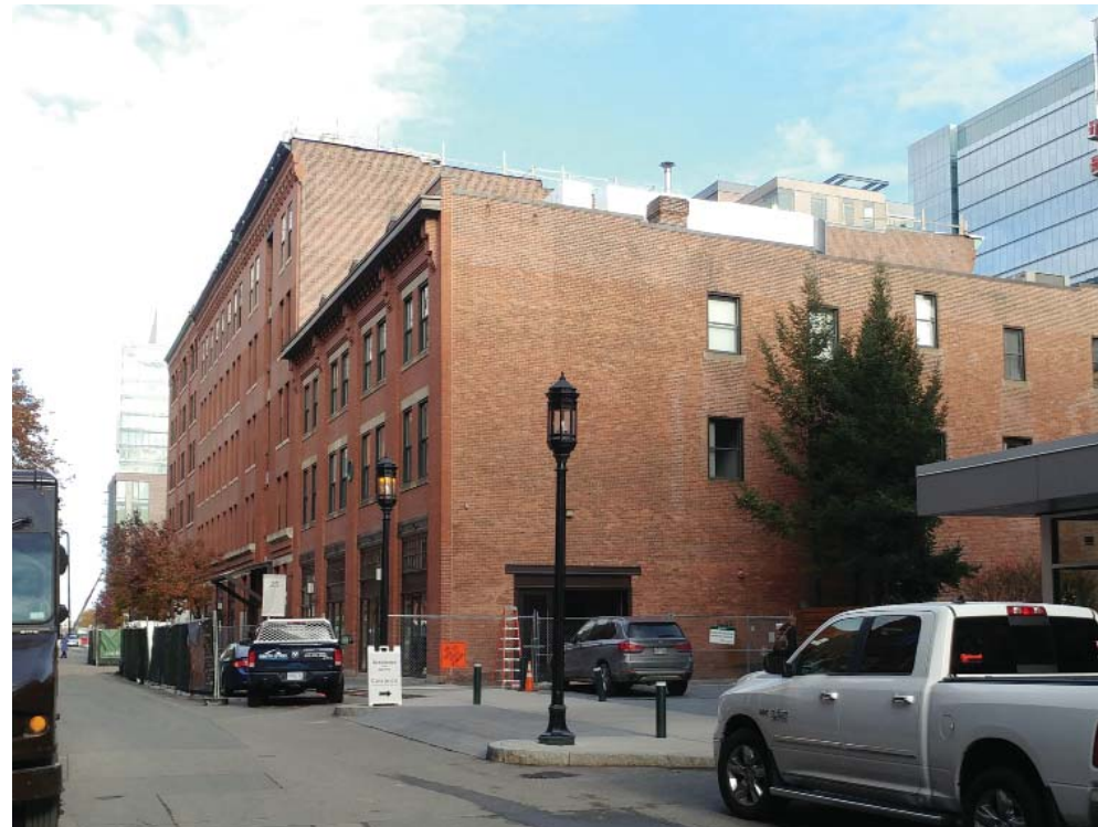
STREET VIEW APPROACHING ON RIGHT
