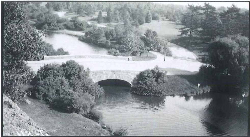
Scarboro Pond Bridge - 1918
