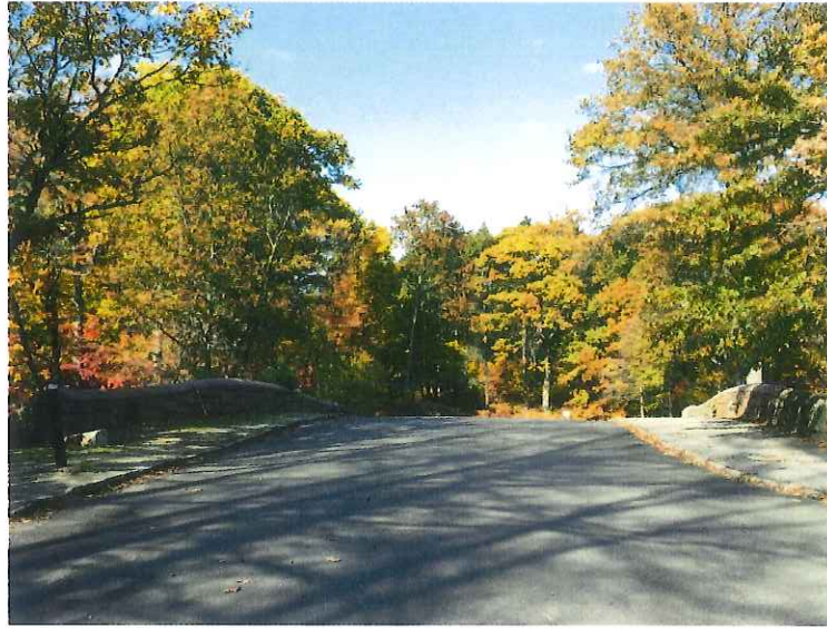
Circuit Drive vehicular bridge over Scarboro Pond (looking north)
