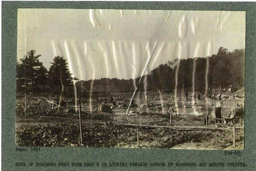
Making of depression for pond
