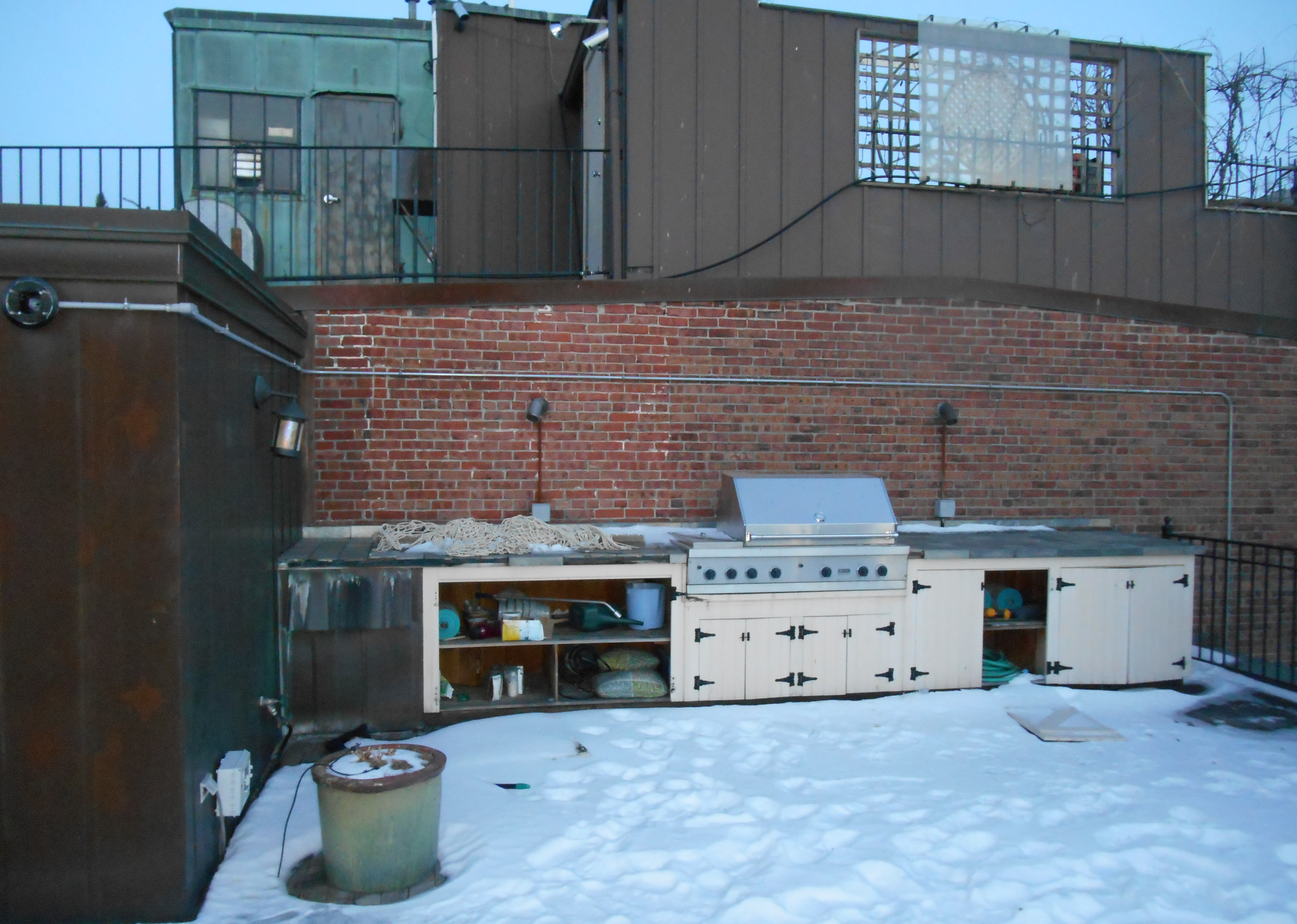
13 COMMONWEALTH AVE - EXISTING CABINETS
