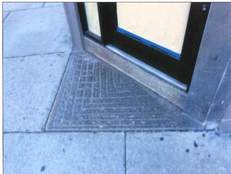
○ ————— Corner - Detail retain granite flooring and step
