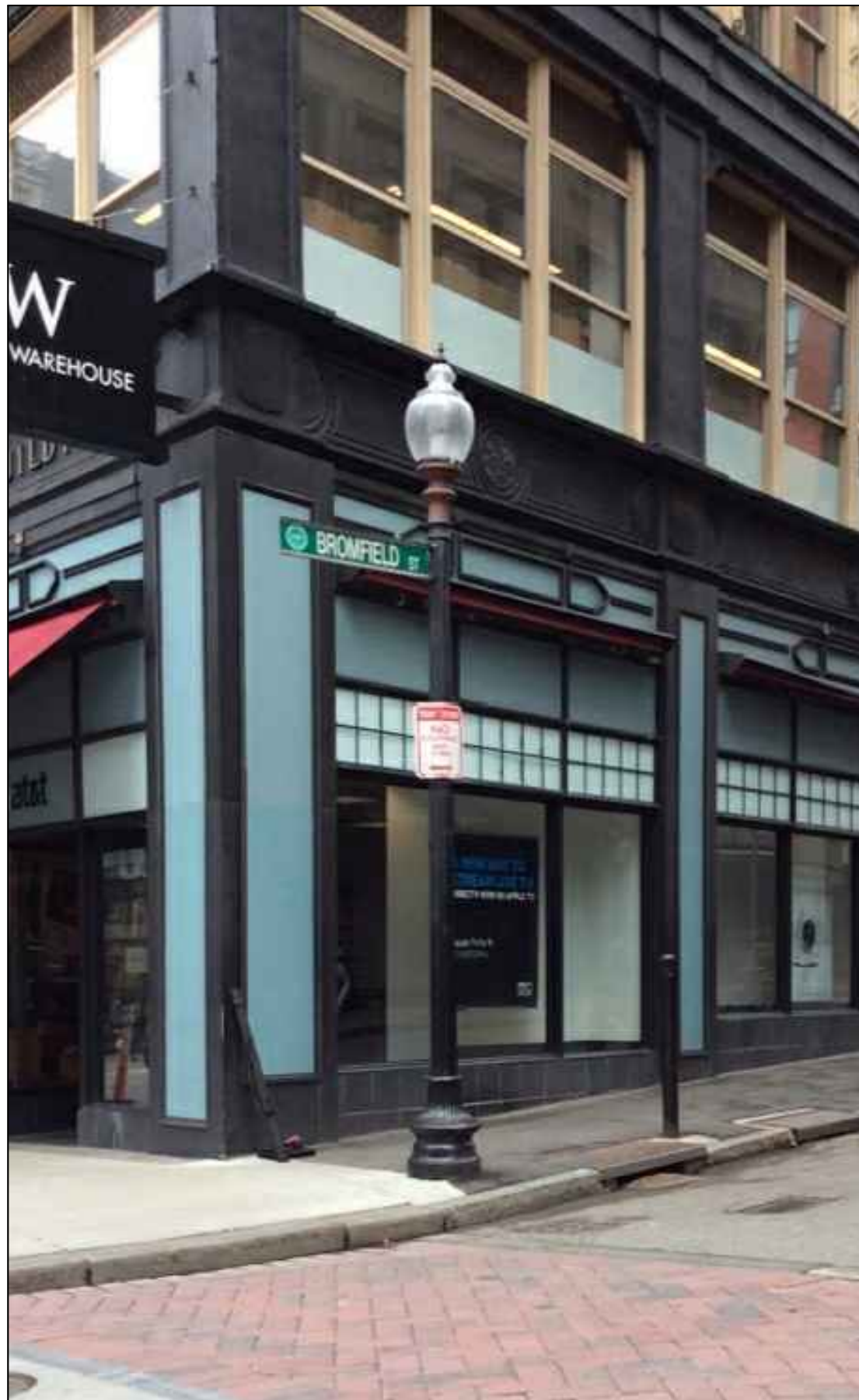
EXISTING PHOTOGRAPHIC VIEW
