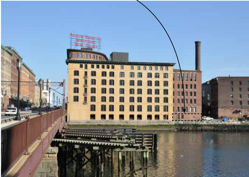
253 Summer Street view from Summer Street Bridge across Fort Point Channel
