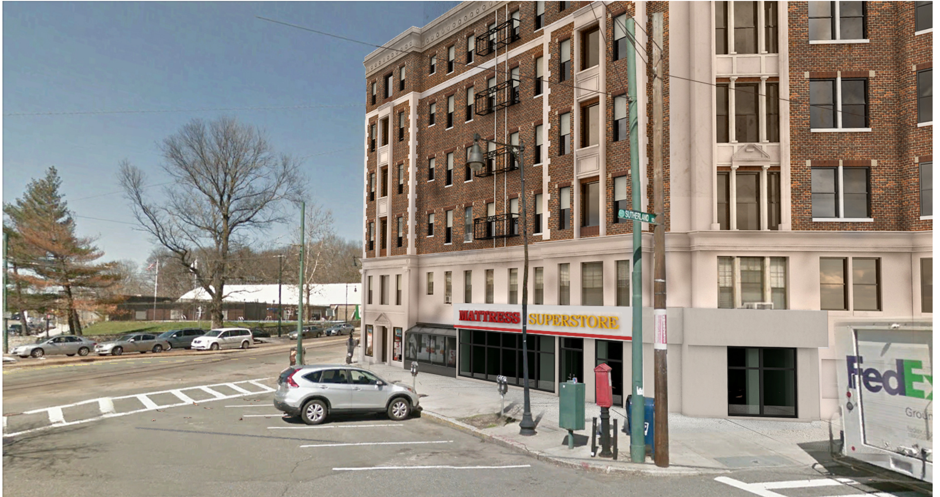
1962 Beacon Street Boston, MA 02135 March 8, 2018
