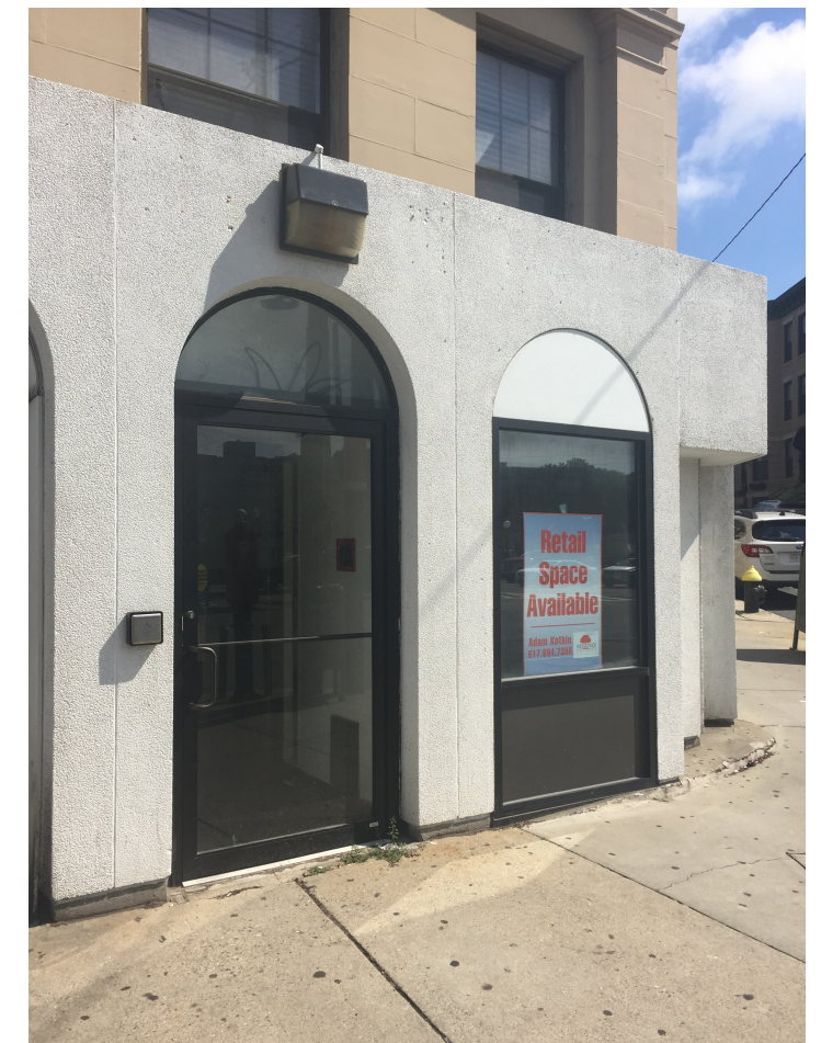
1962 Beacon Street Boston, MA 02135 March 8, 2018
