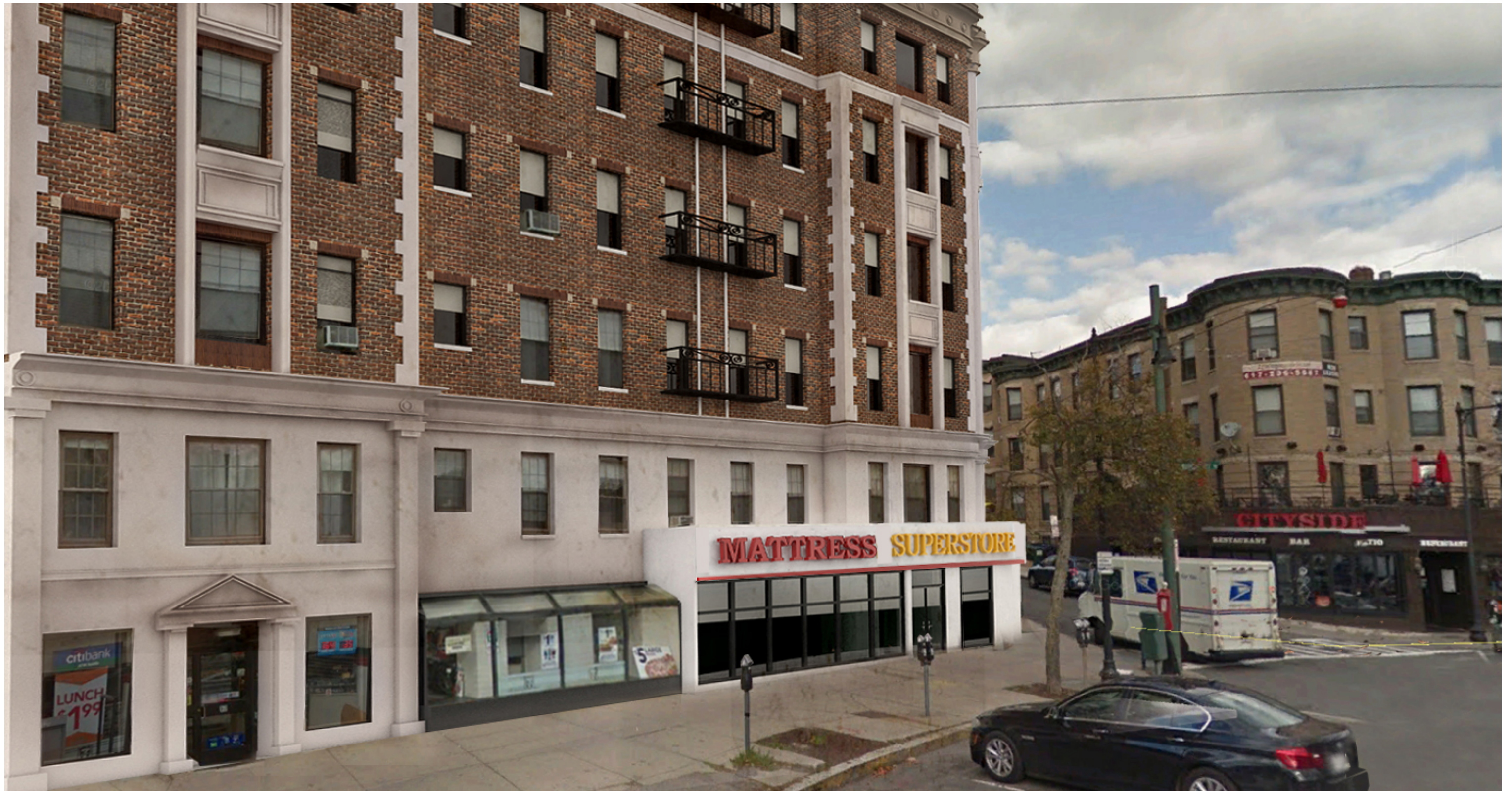
1962 Beacon Street Boston, MA 02135 March 8, 2018
