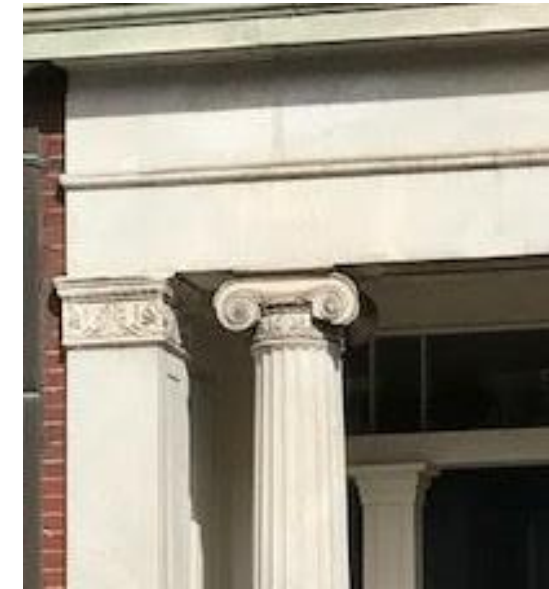
5 COLUMNS, PILASTERS, ENTABLATURE WHITE MARBLE
