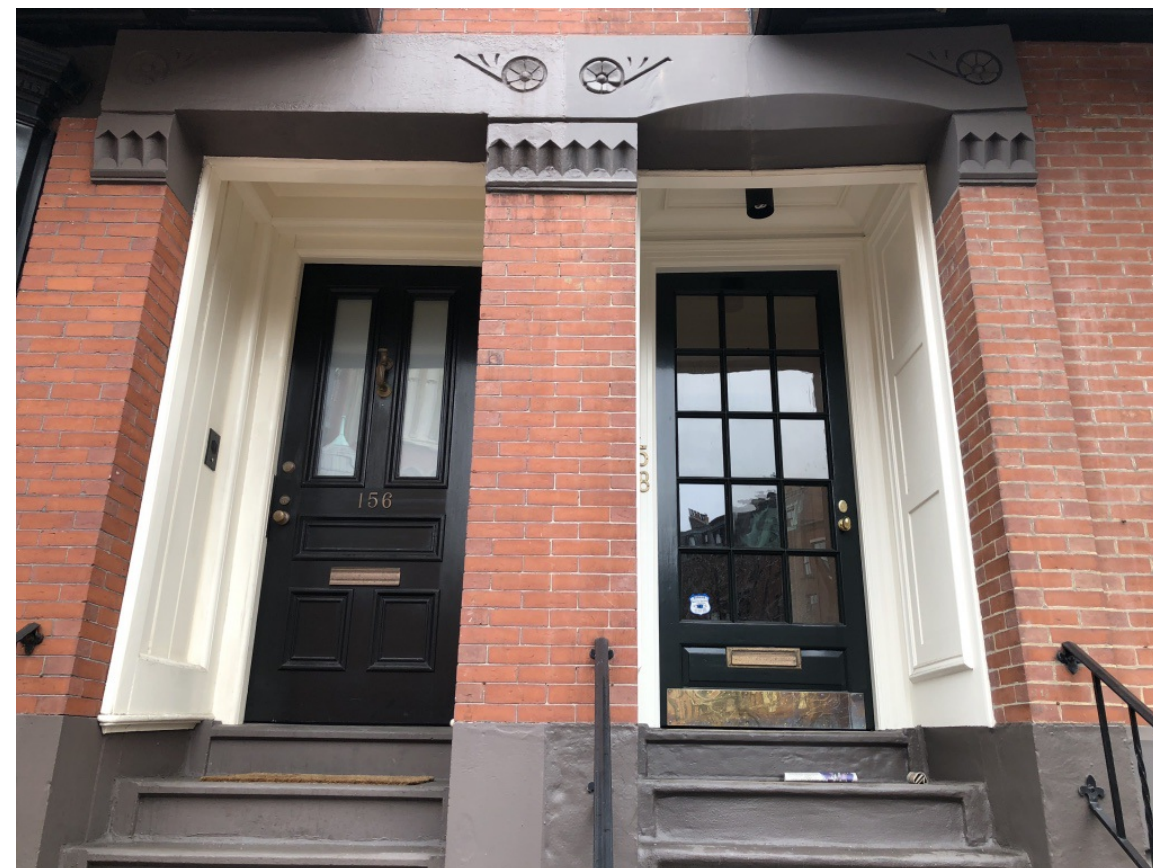
ENTRY DOOR OF 158 AND 156
