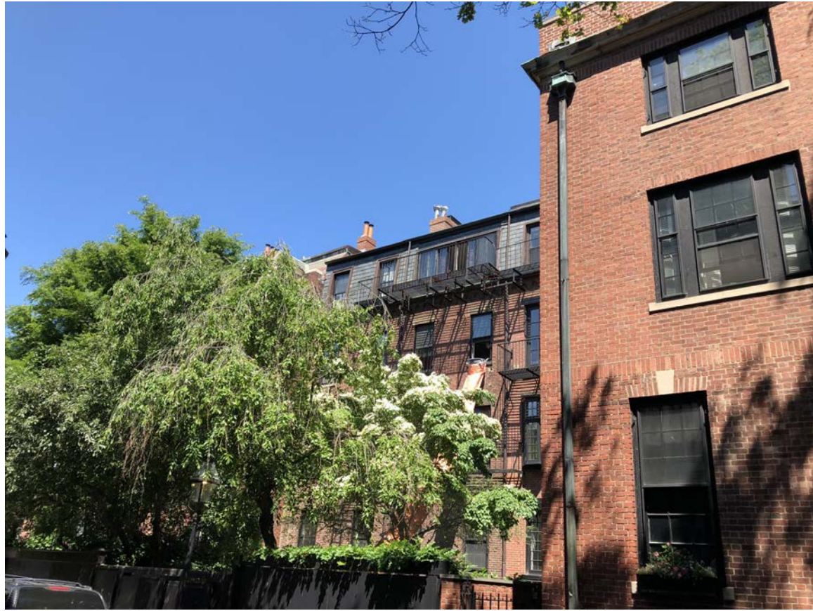
VIEW FROM LIME STREET
