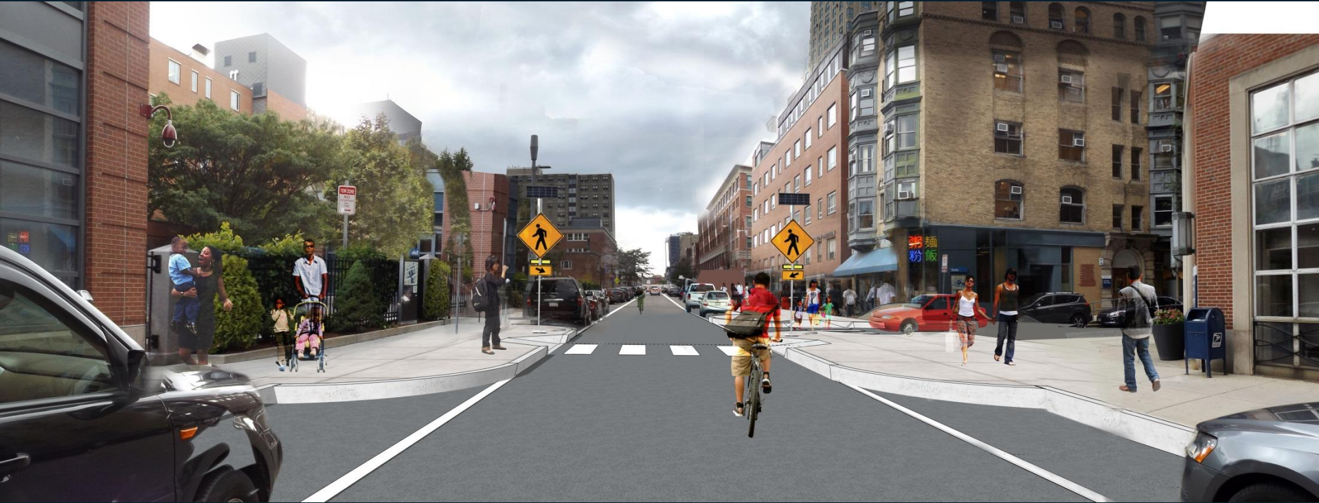
Rendering of curb extensions and signs with lights at Harrison Ave and Bennet St.
