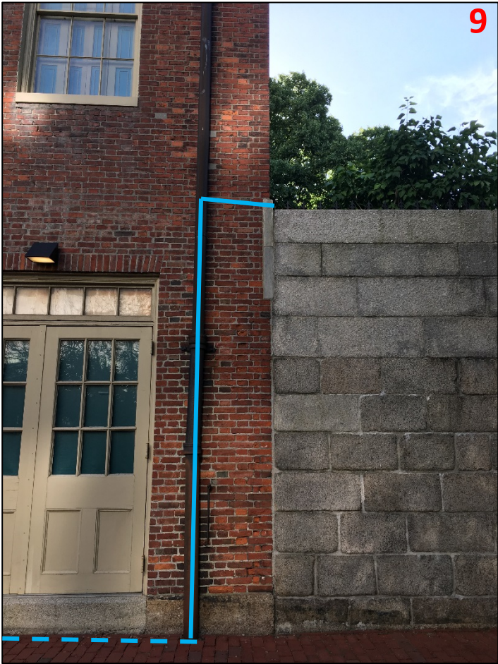
Images above and to left: Photos showing the route of the proposed irrigation line from the faucet next to the staff entrance, down below the brick walkway (buried length indicated in dashed line), up the back of the downspout, and then spanning an approximately 2' width to the edge of the wall of the terrace.
