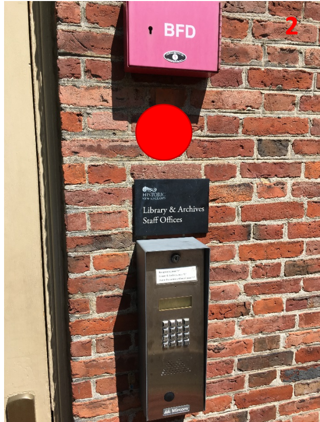
Photo 1 (above) and photo 2 (below), showing the staff entrance and proposed location of the security camera on this elevation (indicated with red dot). Wiring would be run either from behind camera or up from existing call box. Camera would be Axis M3027-PVE Network Camera (see cut sheets on following pages.)
