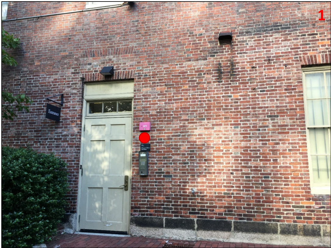
Photo 1 (above) and photo 2 (below), showing the staff entrance and proposed location of the security camera on this elevation (indicated with red dot). Wiring would be run either from behind camera or up from existing call box. Camera would be Axis M3027-PVE Network Camera (see cut sheets on following pages.)
