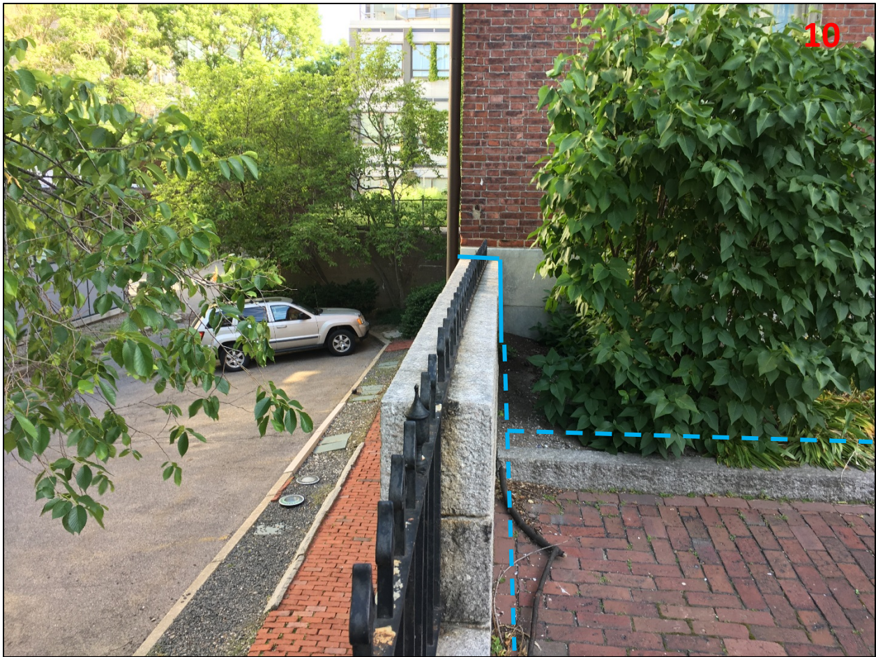
Image above: Photo showing the route of the proposed irrigation line from the top of the terrace side wall, down the interior edge of the terrace side wall, and then buried to service plantings (buried lengths indicated in dashed lines).
