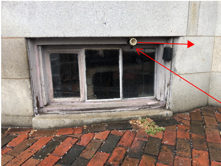
Close-up of window to be replaced
