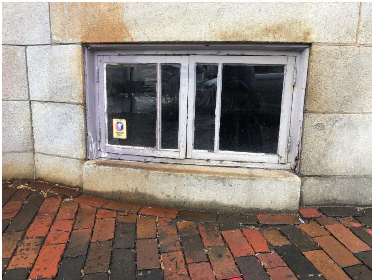
Close-up of other window to be replaced
