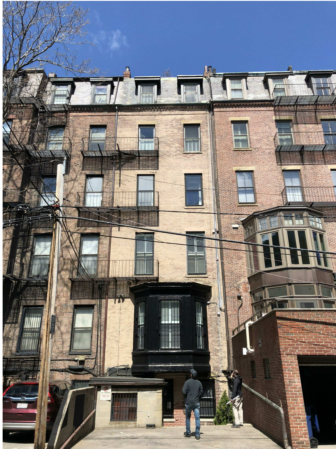
EXISTING REAR FACADE
