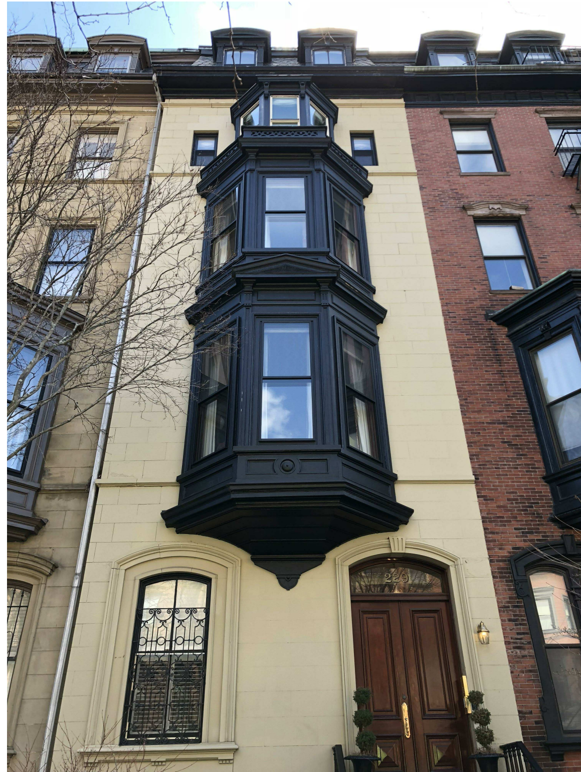
EXISTING FRONT FACADE
