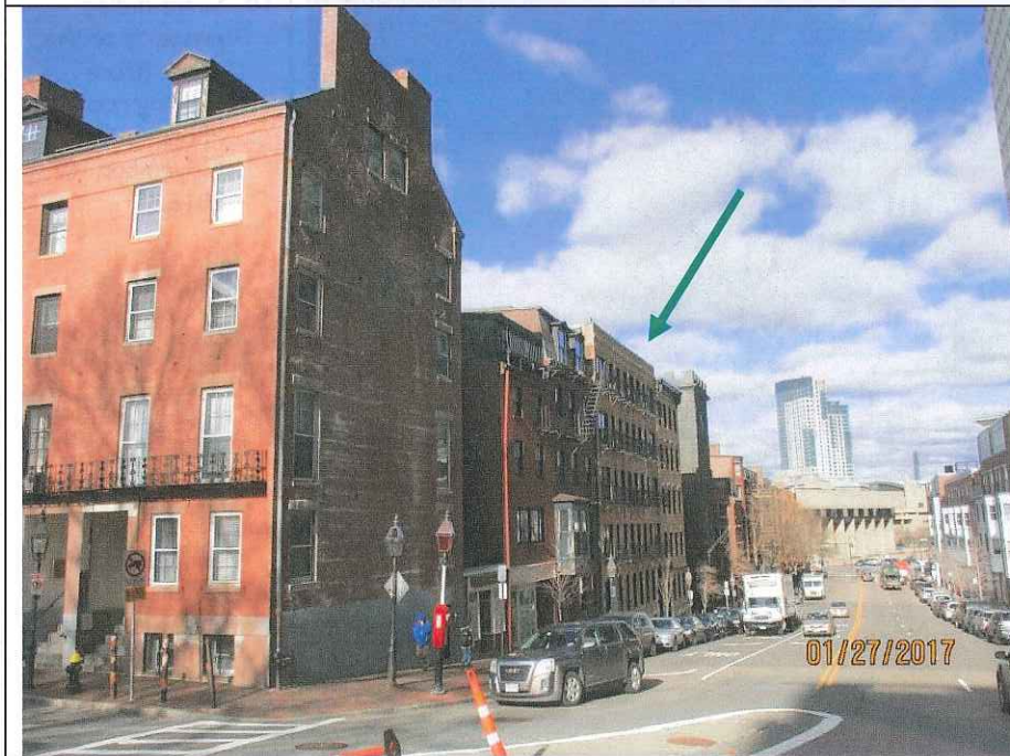
12. Context view north-northwest toward Subject Property (green arrow). Photo taken January 27, 2017.
