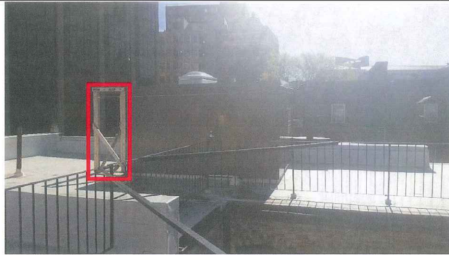
5. View southeast toward location of proposed Sector B antennas within proposed fiberglass chimney (left of penthouse) and proposed steel equipment platform (right of penthouse). Photo taken November 10, 2016.
