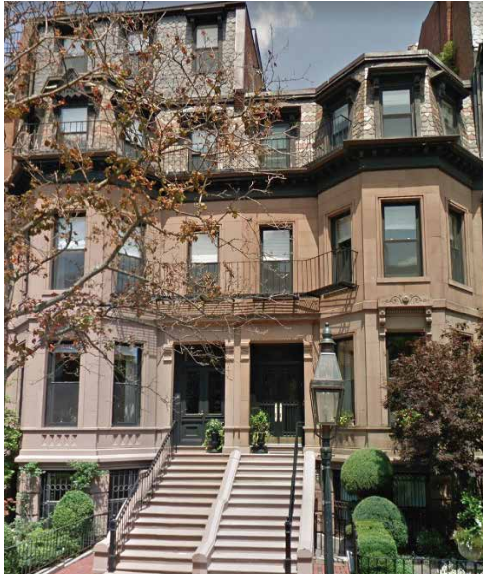
Existing Front Facade Photo
