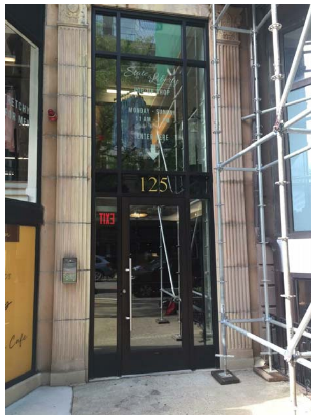
EXISTING MAIN ENTRY VIEW:
