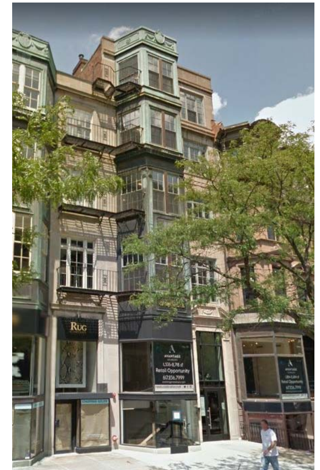
EXISTING FULL BUILDING VIEW:
