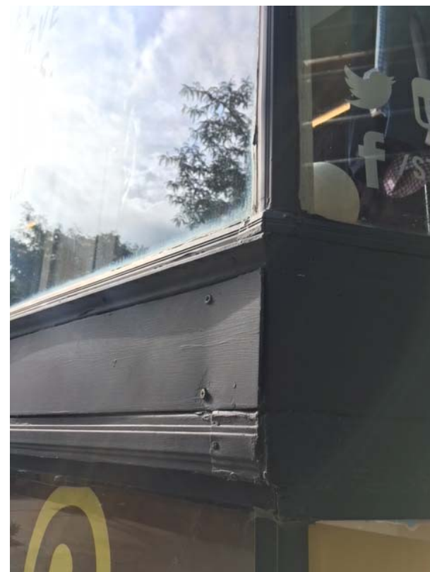
EXISTING SIGN MOUNTING CONDITION:
