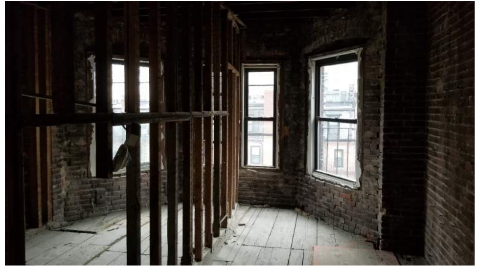
4th floor bay, right side
