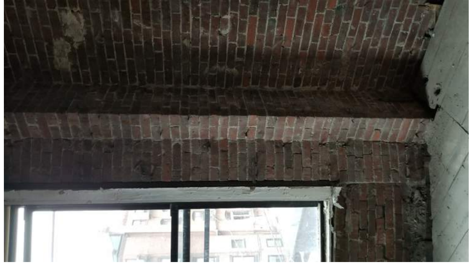
2nd floor bay
