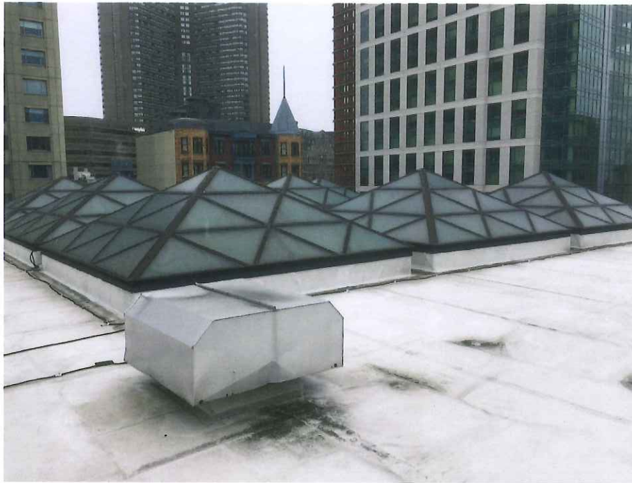
Figure 8: Johnson Building – Skylights
