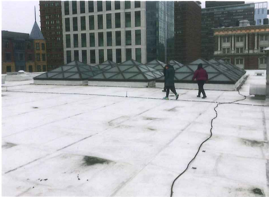
Figure 20: Johnson Building – PVC Roof
