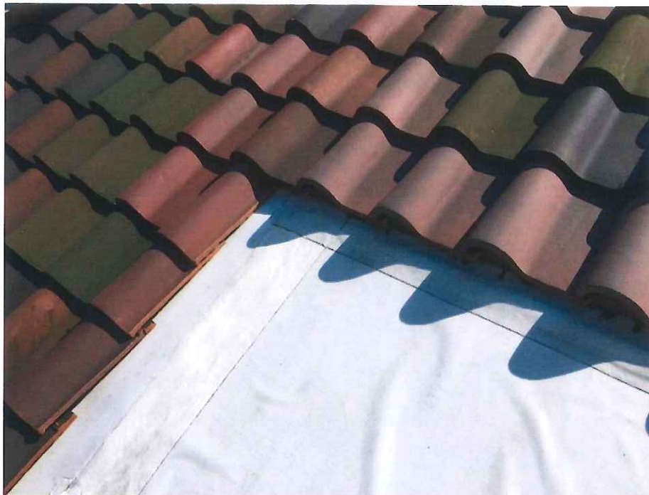
Figure 17: McKim Building – Tile and PVC Roof Intersection
