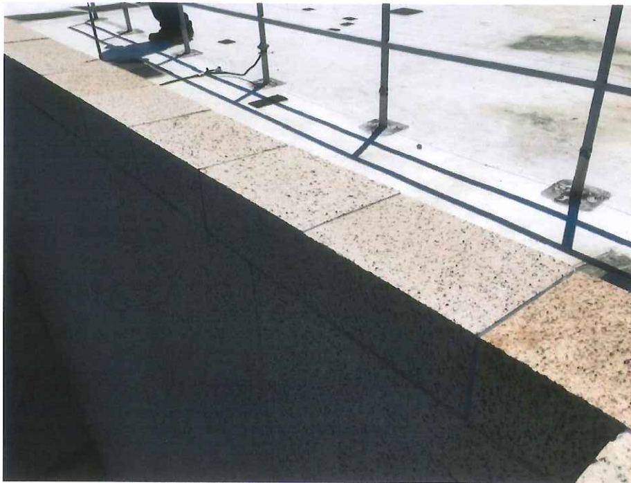
Figure 22: Johnson Building – Granite Coping
