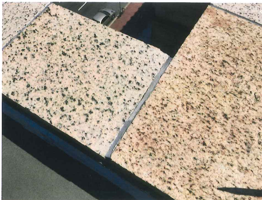
Figure 23: Johnson Building – Granite Coping
