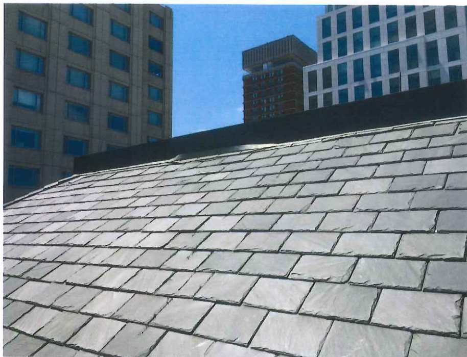
Figure 12: Johnson Building – Slate Roof
