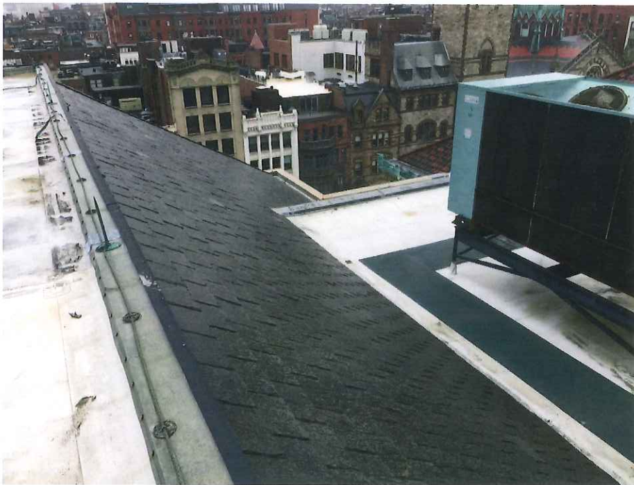
Figure 15: Johnson Building – Slate Roof
