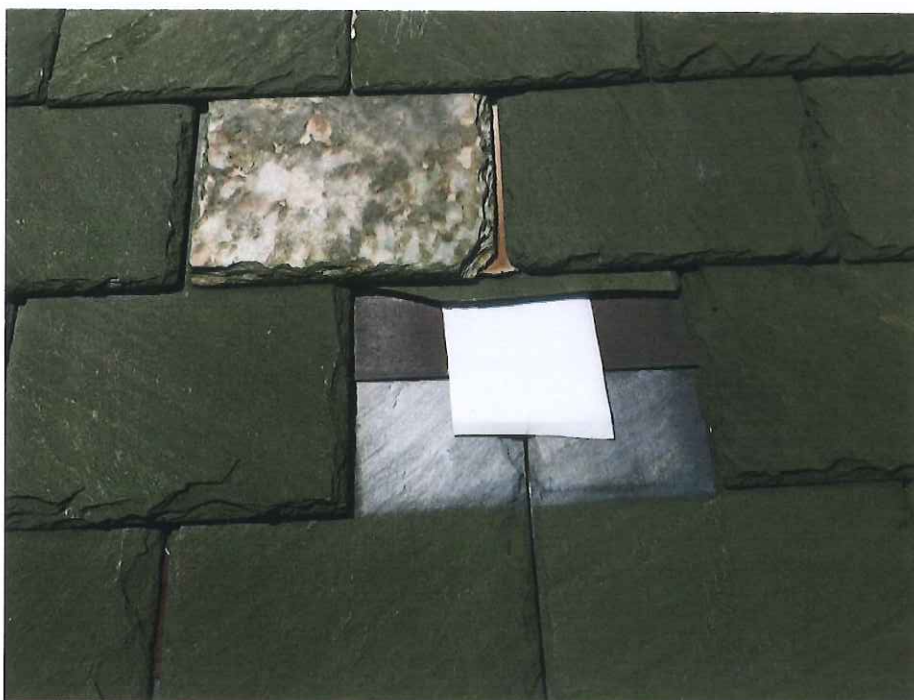
Figure 13: Johnson Building – Slate Roof
