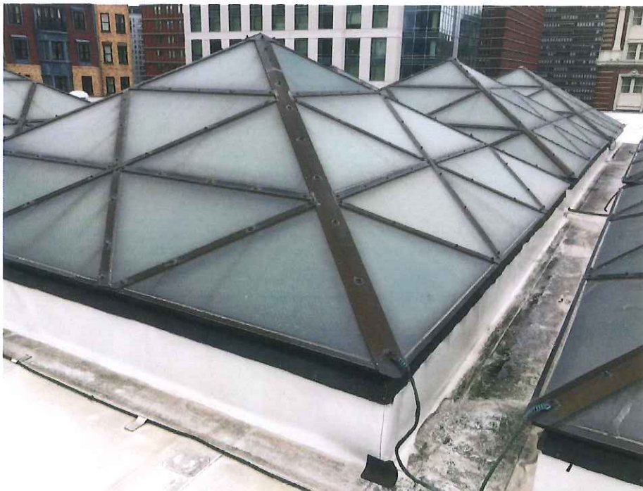
Figure 9: Johnson Building – Skylights
