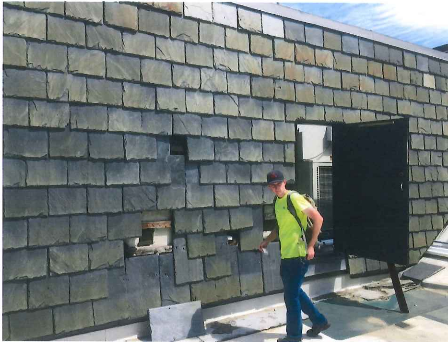
Figure 14: Johnson Building – Slate Screen Wall
