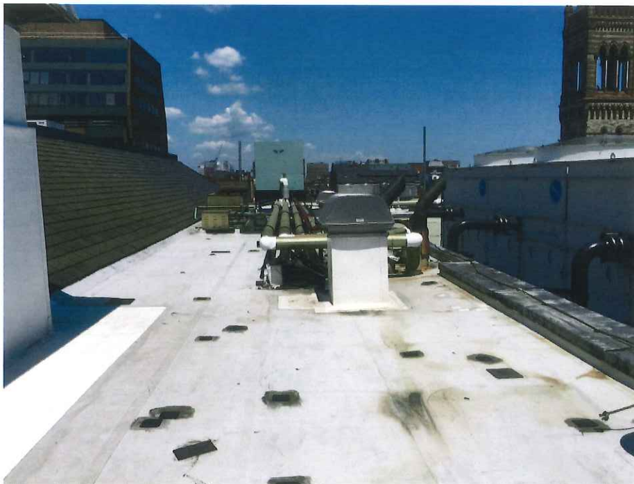
Figure 21: Johnson Building – PVC Roof
