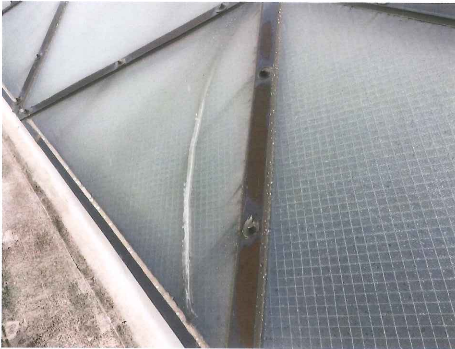
Figure 10: Johnson Building – Skylights
