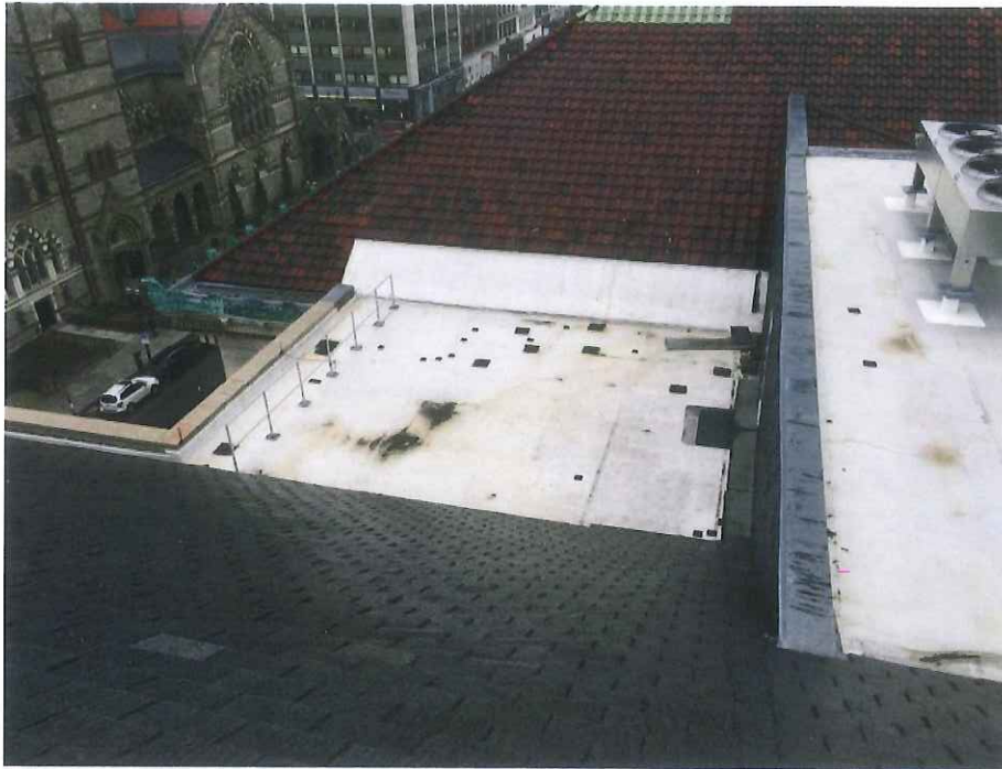
Figure 16: McKim Building – Tile and PVC Roof Intersection
