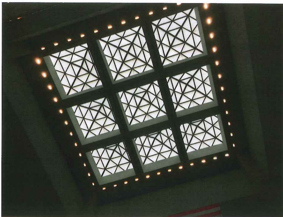
Figure 11: Johnson Building – Skylights at Interior Atrium
