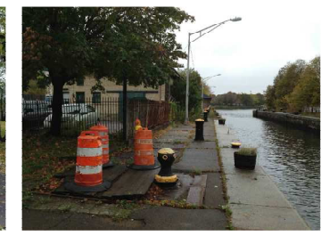
MOORING BOLLARDS AND CLEATS
