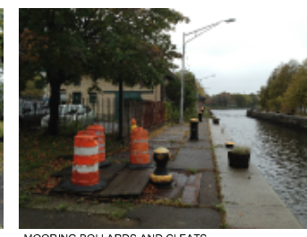
MOORING BOLLARDS AND CLEATS
