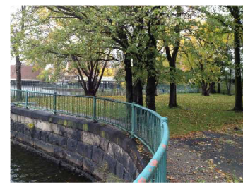
ESPLANADE GUARDRAIL (CHARLES RIVER STANDARD)
