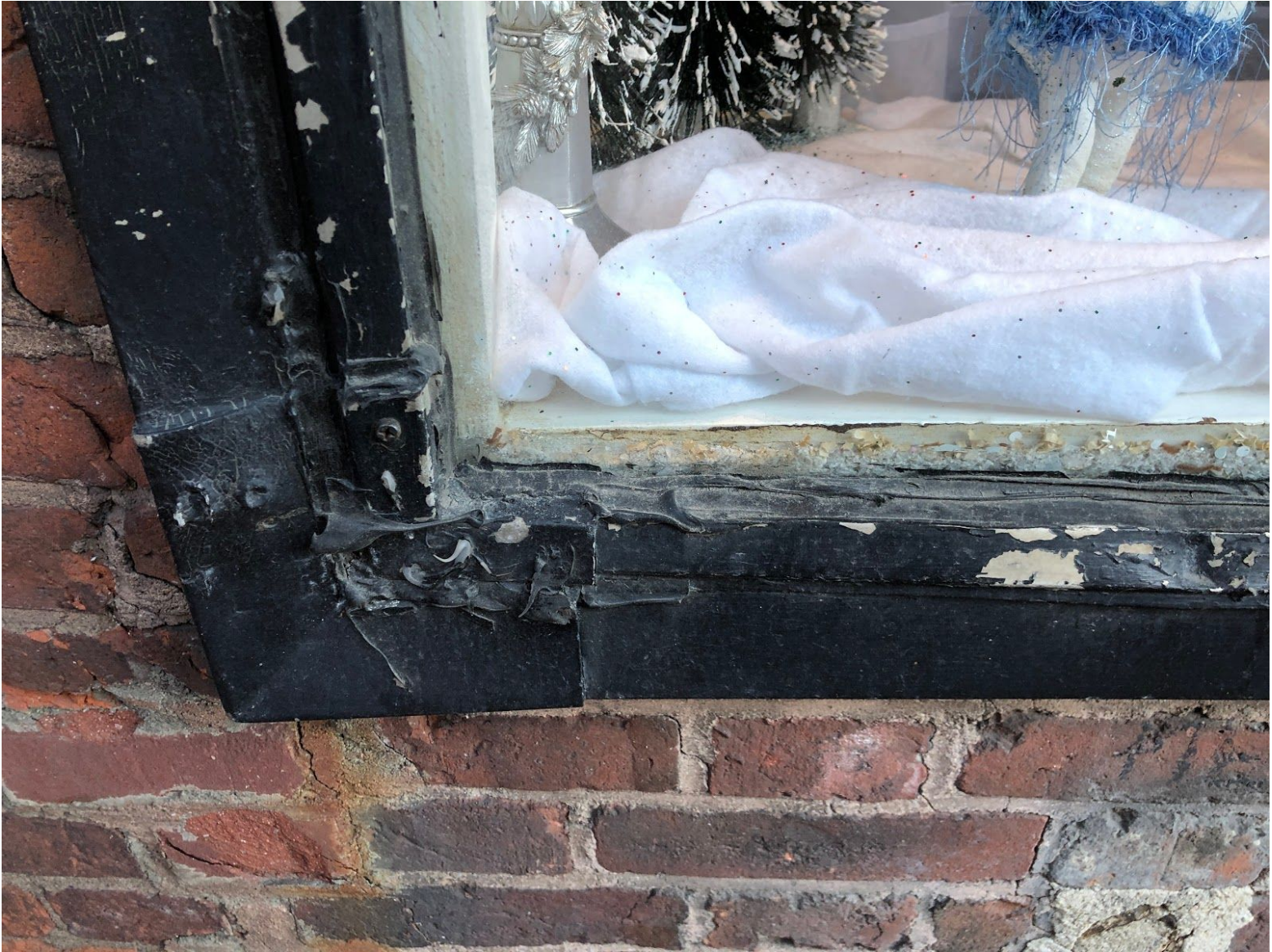
81 Charles Street exterior window, lower left corner detail
