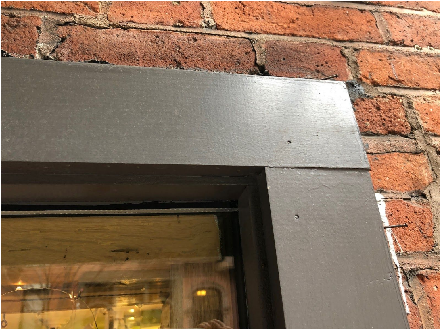
83 Charles Street exterior window, upper right hand corner detail:
