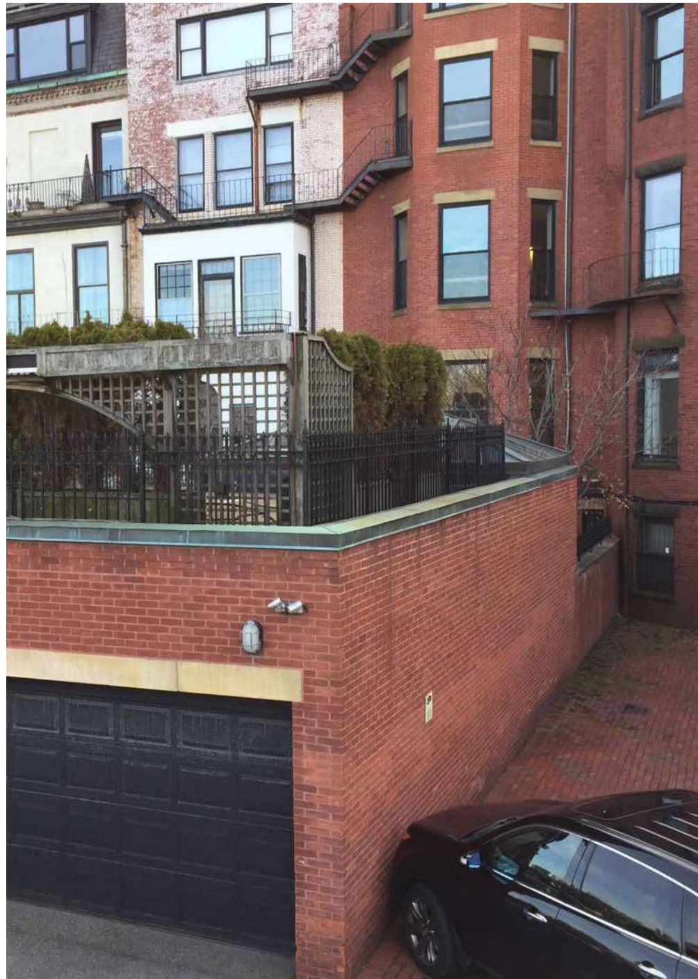
Modifications to rear courtyard would not be visible from the right-of-way or pedestrian bridge
