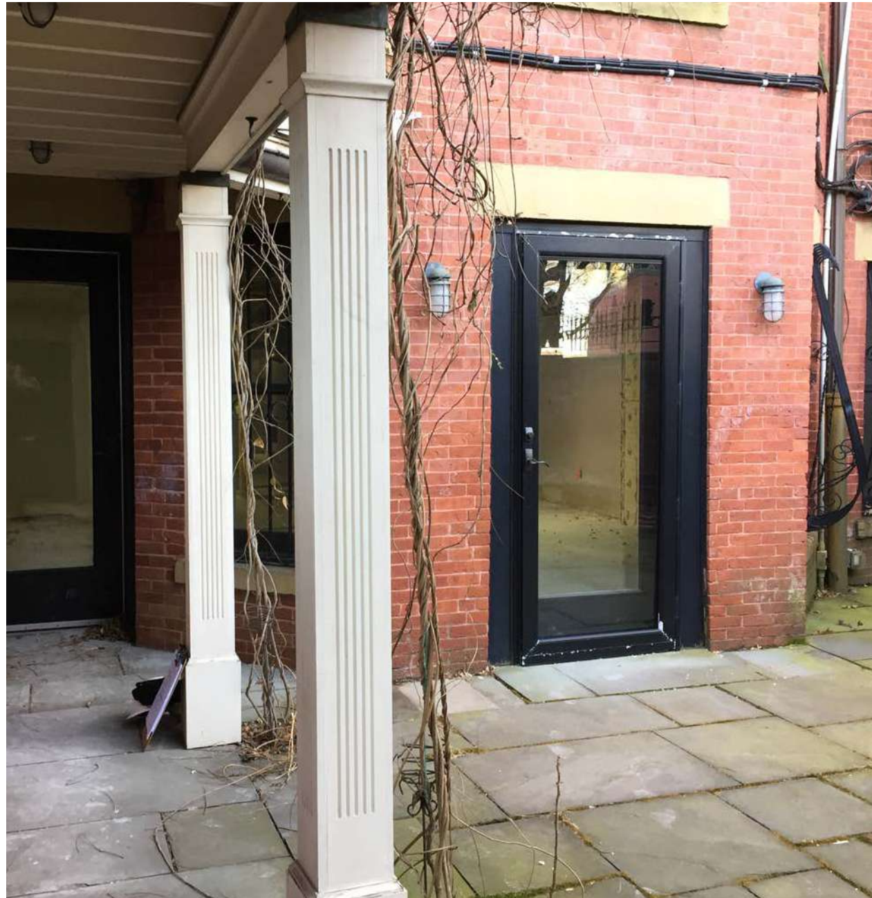
Replace outswing patio door @ rear courtyard; • no change to existing opening
