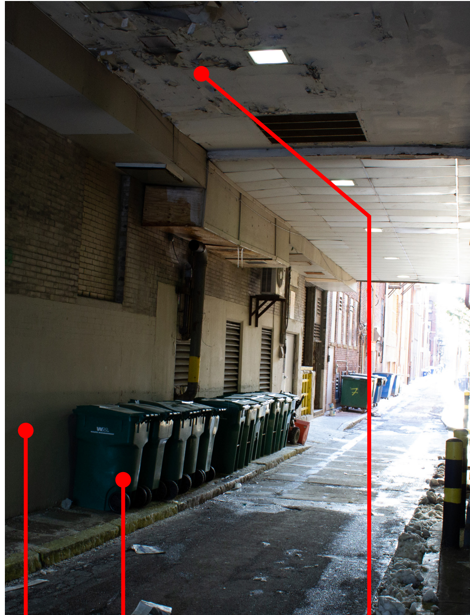
DUMPSTERS TO BE REMOVED
