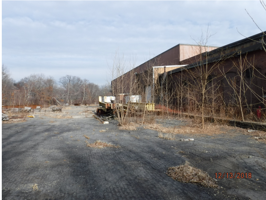
Photograph 1: Rear of the property behind the existing building.
