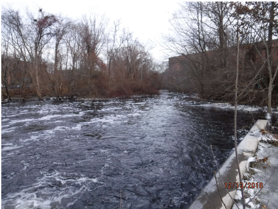
Photograph 8: View of Mother Brook, looking downstream toward proposed work areas.
