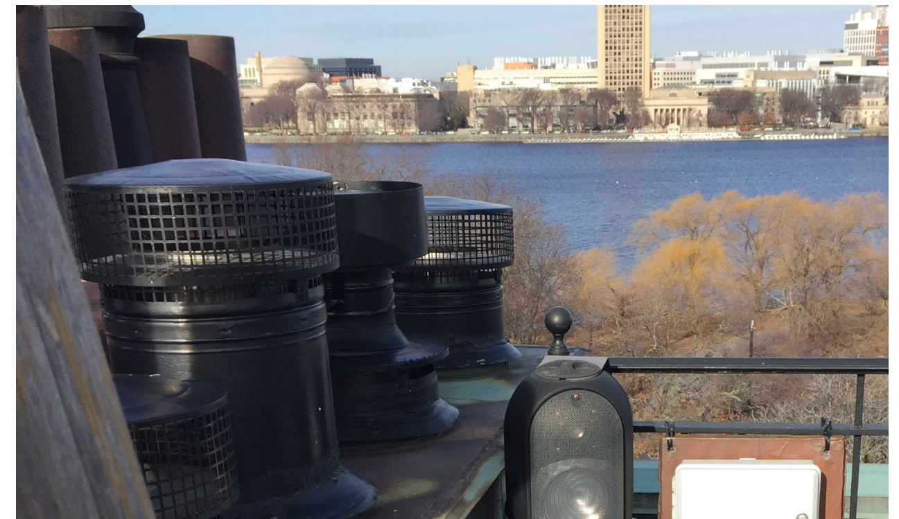
EXISTING CHIMNEY FLUE CAPS
