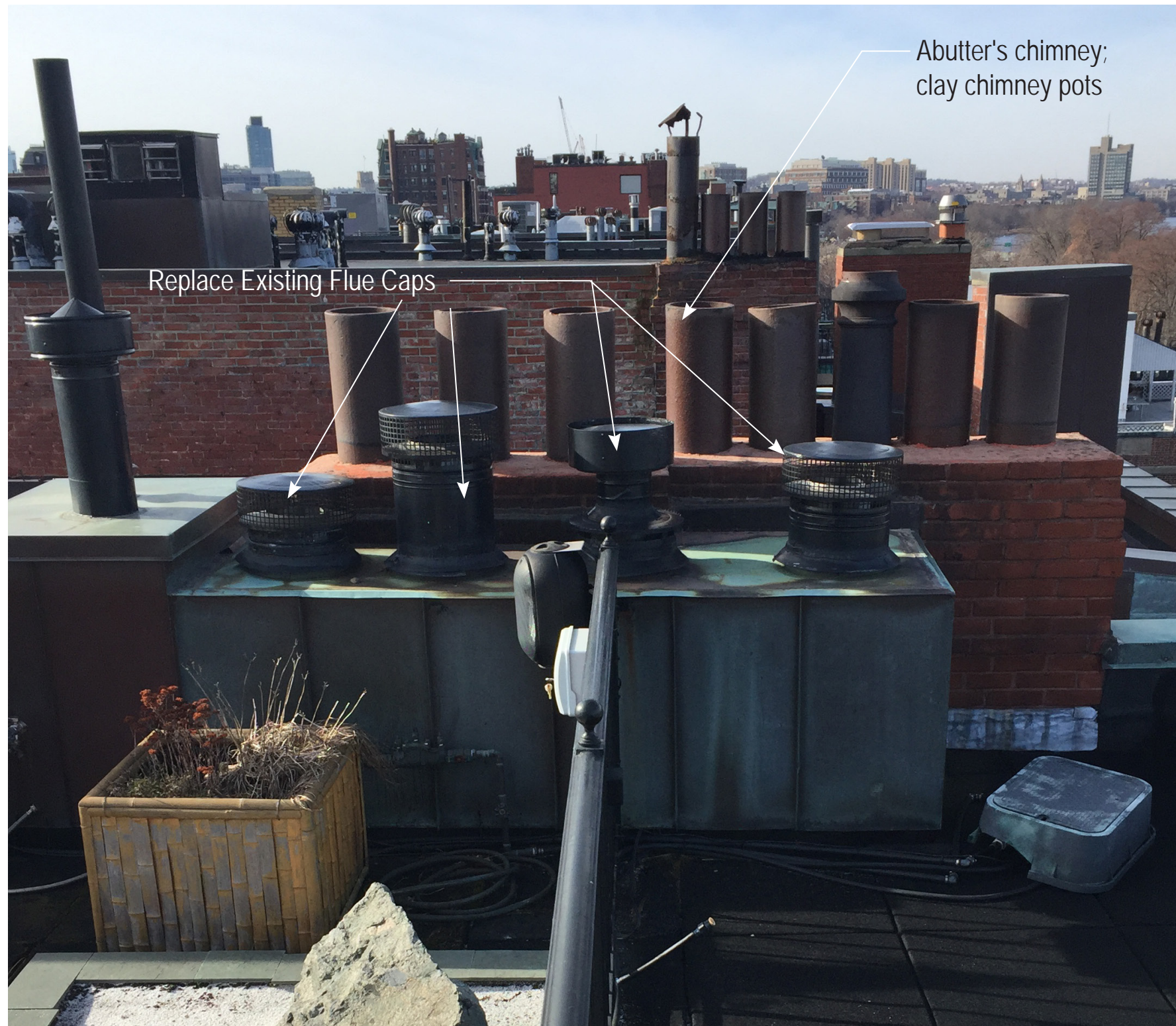
EXISTING CHIMNEY FLUE CAPS
