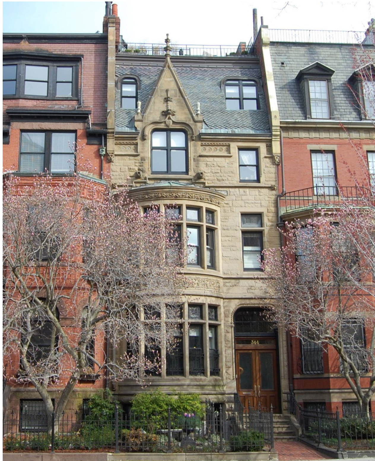
344 BEACON - FRONT FACADE
