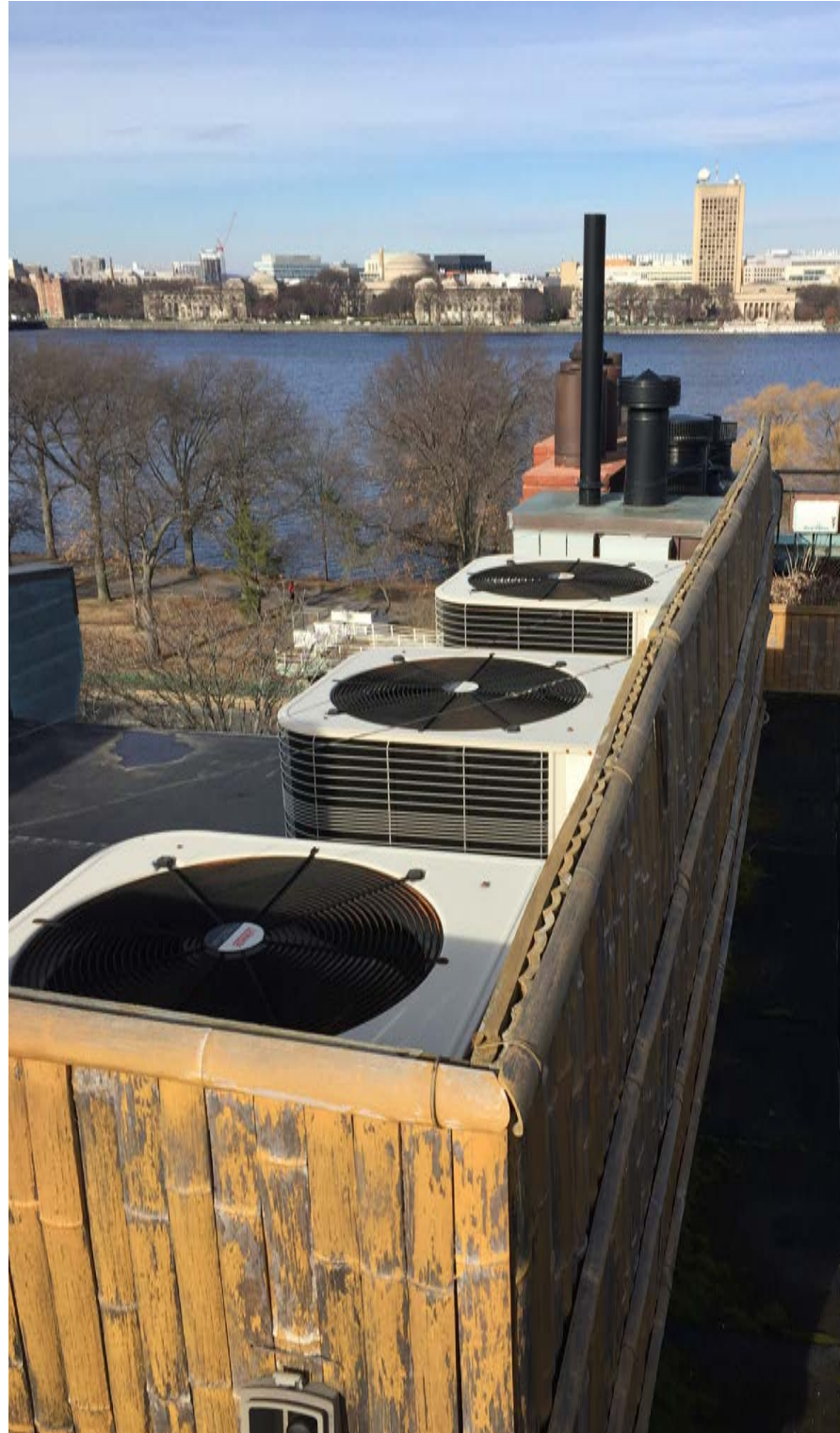
EXISTING MECHANICAL EQP. SCREEN WALL
