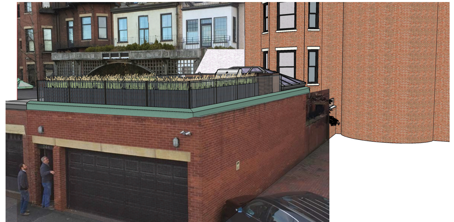
VIEW FROM PEDESTRIAN BRIDGE
