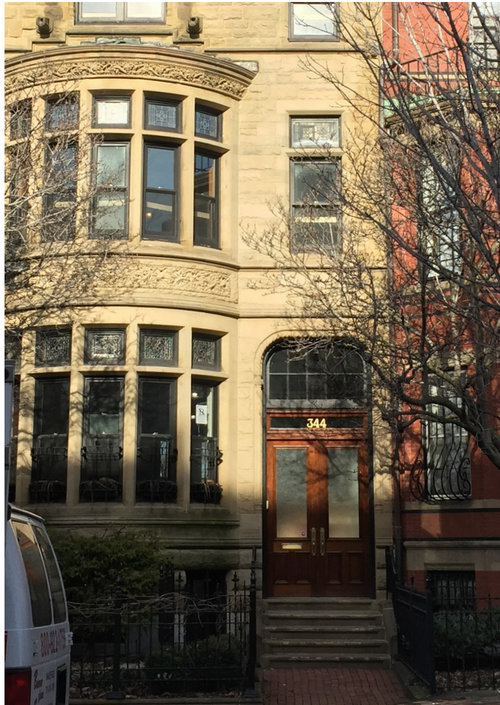
EXISTING ENTRY DOOR
