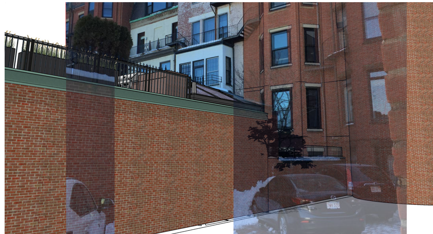
VIEW FROM BACK STREET
